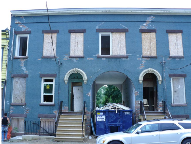
Photo of the front of the building, showing that the building was not occupied
