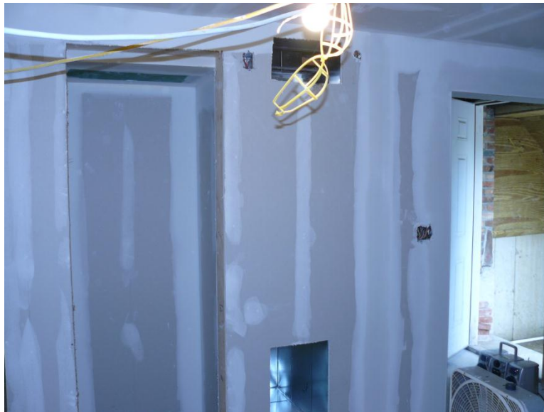
Interior photo of a lower level apartment, which was not complete
