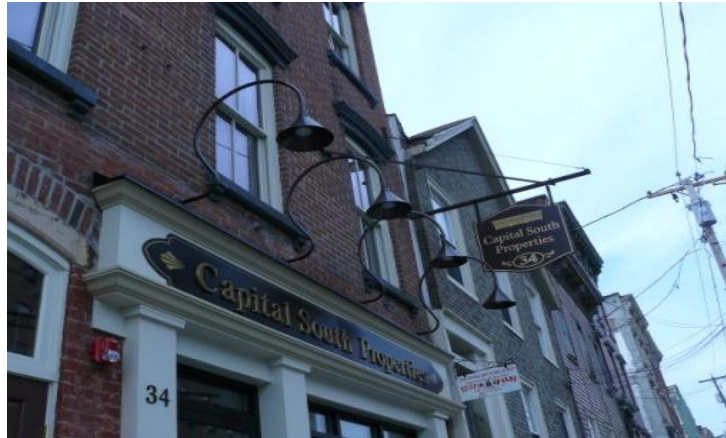
This photo shows that only four goose neck lighting fixtures were installed.
