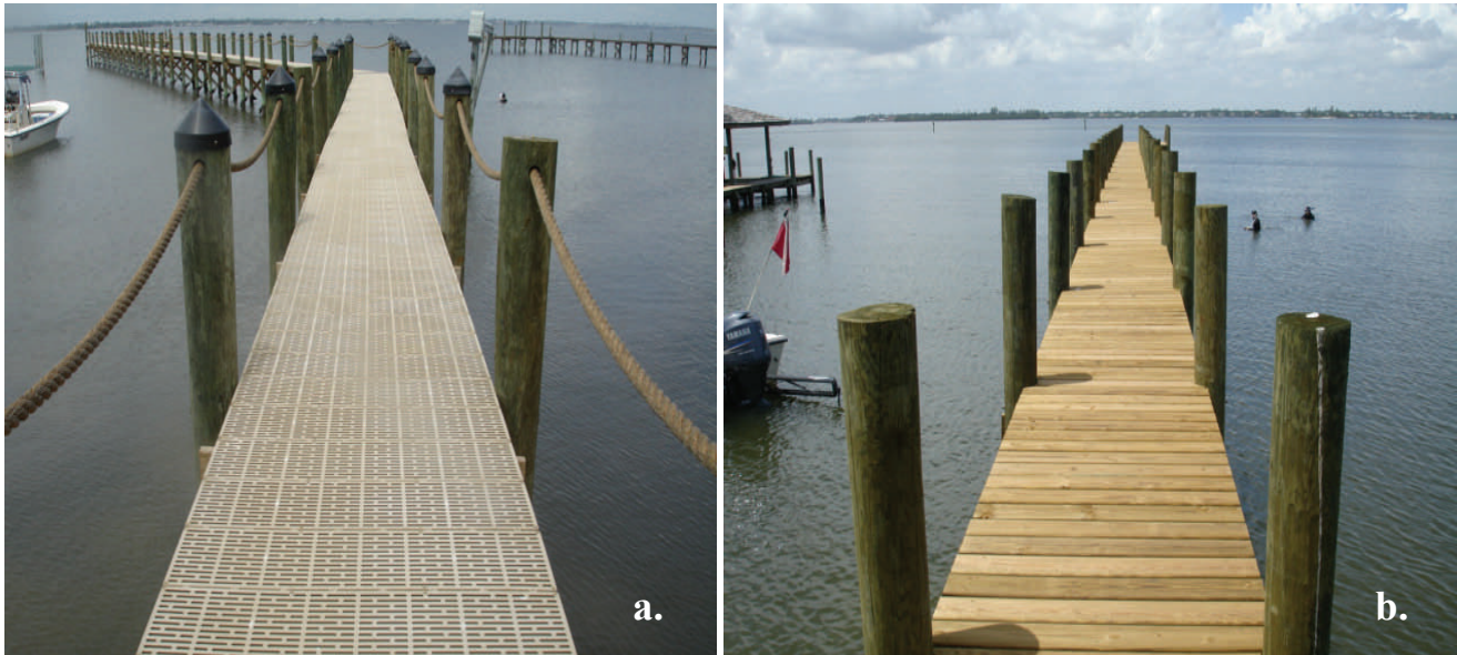
Figure 1. Light transmitting (a) and planked (b) docks.
