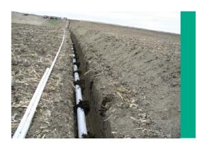
Switching from gravity irrigation to a sub-surface drip irrigation can reduce the amount of water applied to fields by one third.
