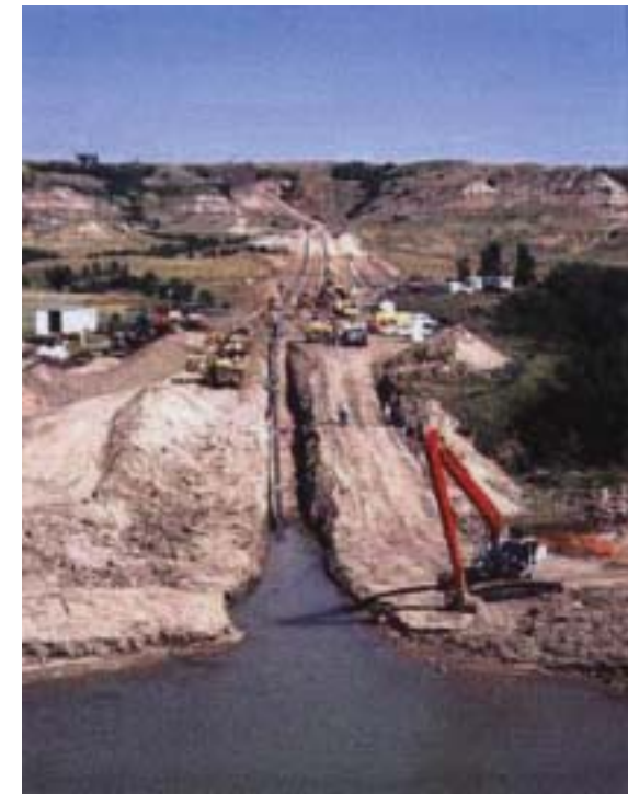
Picture of CO 2 pipeline installation
