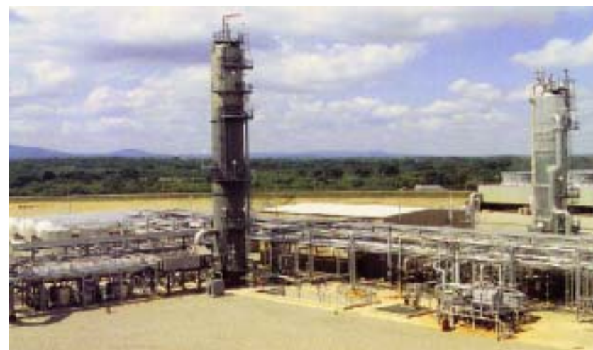
IMC Chemicals \text{CO}_2 Capture Plant
