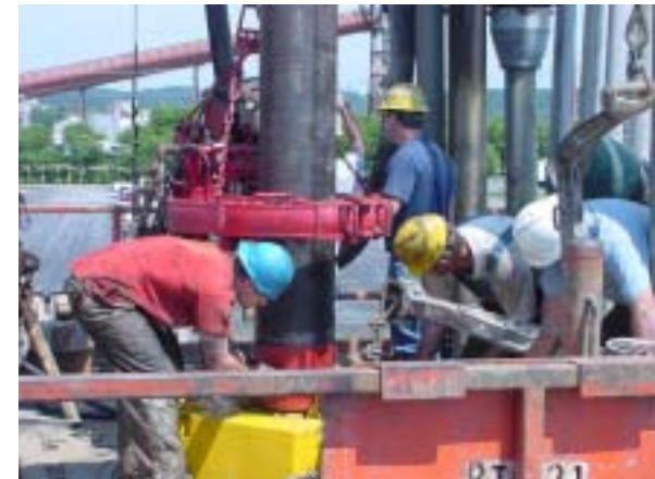
Mountaineer – Installation of 13-inch Casing
