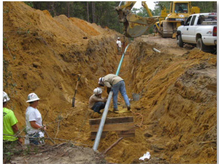
Figure 3 - Construction of the CO 2 pipeline for the Plant Barry Site
