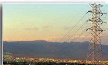
Electric tower, Mexico.
