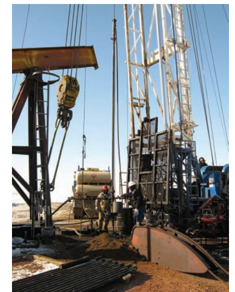
Preparation of the injection well for the PCOR Partnership's huff 'n' puff test.
