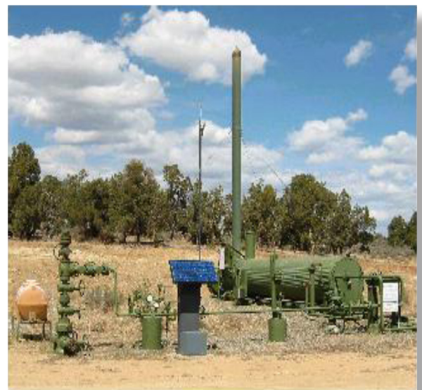
Figure 2: CO 2 injector well at the Allison Unit.
