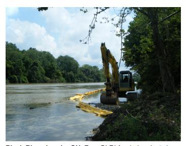
**Black River, Lorain, OH.** Four GLRI-funded projects in the Black River Area of Concern include the construction of 5000+ linear ft. of fish habitat shelves, approx. 1500 ft. of riverbank stabilization and restoration, the removal of 45,000 cubic yards of steel slag, the restoration of 2.3 acres of riparian habitat, the engineering and design of additional in-stream and bank restoration, and the treatment of invasive species.
