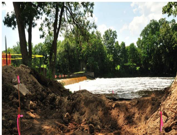
A fish passage project on the Milwaukee River.
