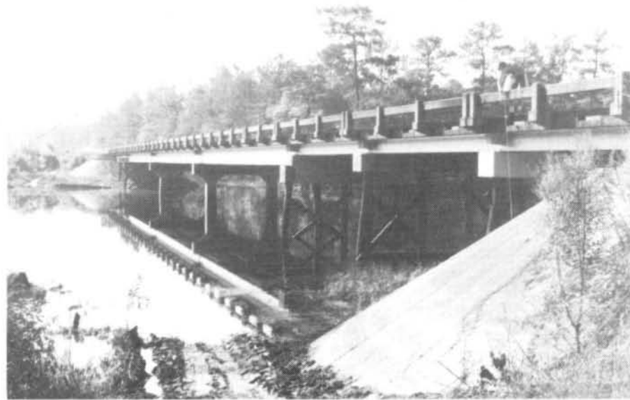
FIGURE 9 - N. C. 904 HIGHWAY BRIDGE (R.M. 102.1)
