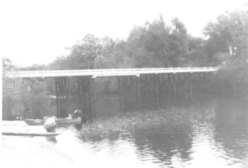
FIGURE 3 - S. C. SECONDARY 105 HIGHWAY BRIDGE (R.M. 62.7)
