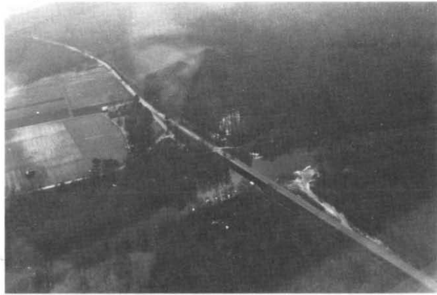
FIGURE 2 - UTILITY LINE (R.M. 62.7) (S. C. SECONDARY 105 HIGHWAY BRIDGE)
