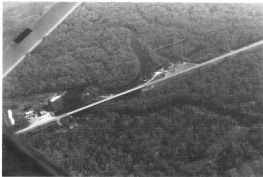
FIGURE 7 - UTILITY LINE (R.M. 85.1) (S. C. 9 HIGHWAY BRIDGE)
