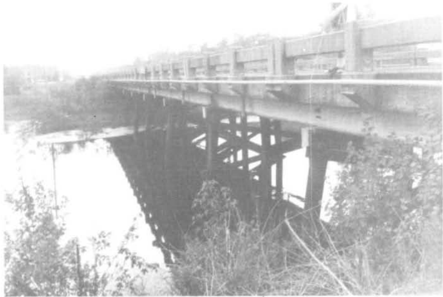
FIGURE 8 - S. C. 9 HIGHWAY BRIDGE (R.M. 85.4)
