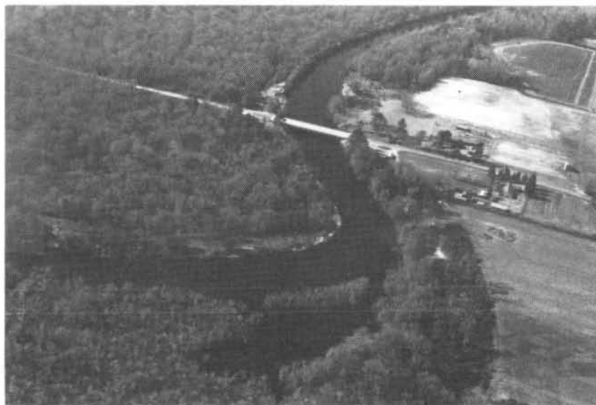
FIGURE 5 - UTILITY LINE (R.M. 70.5) (S. C. SECONDARY 31 HIGHWAY BRIDGE)
