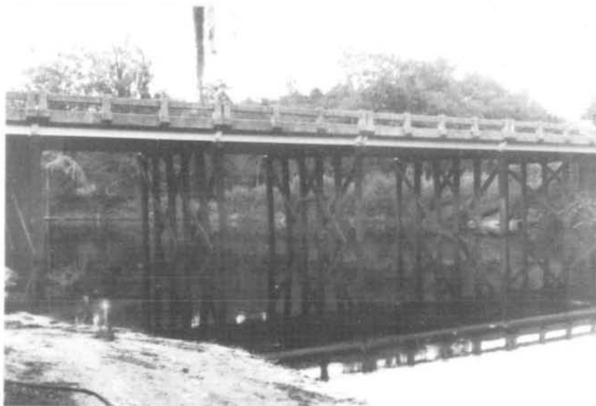
FIGURE 11 - N. C. 130 HIGHWAY BRIDGE (R.M. 118.3)
