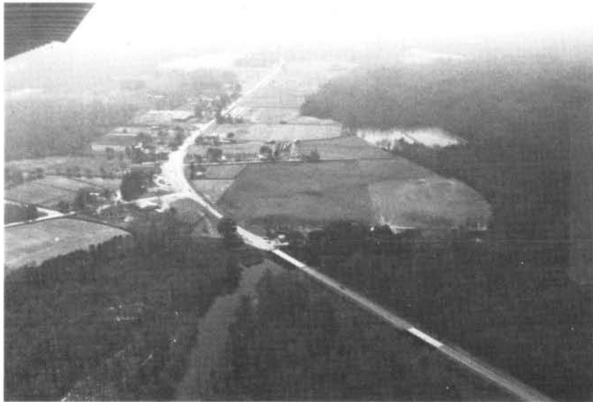
FIGURE 12 - UTILITY LINE (R.M. 118.3) (N. C. 130 HIGHWAY BRIDGE)
