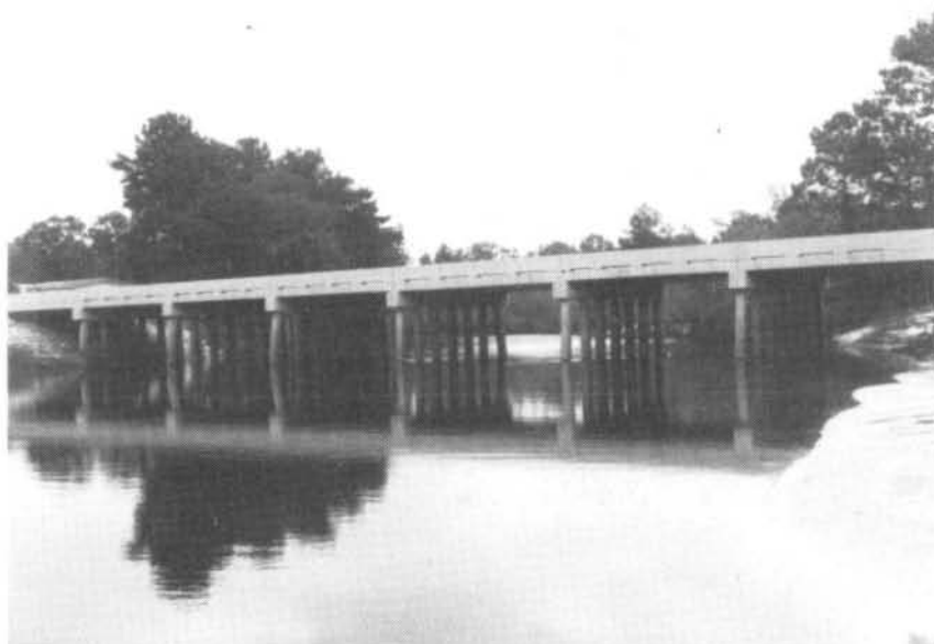
FIGURE 4 - S. C. SECONDARY 31 HIGHWAY BRIDGE (R.M. 70.4)
