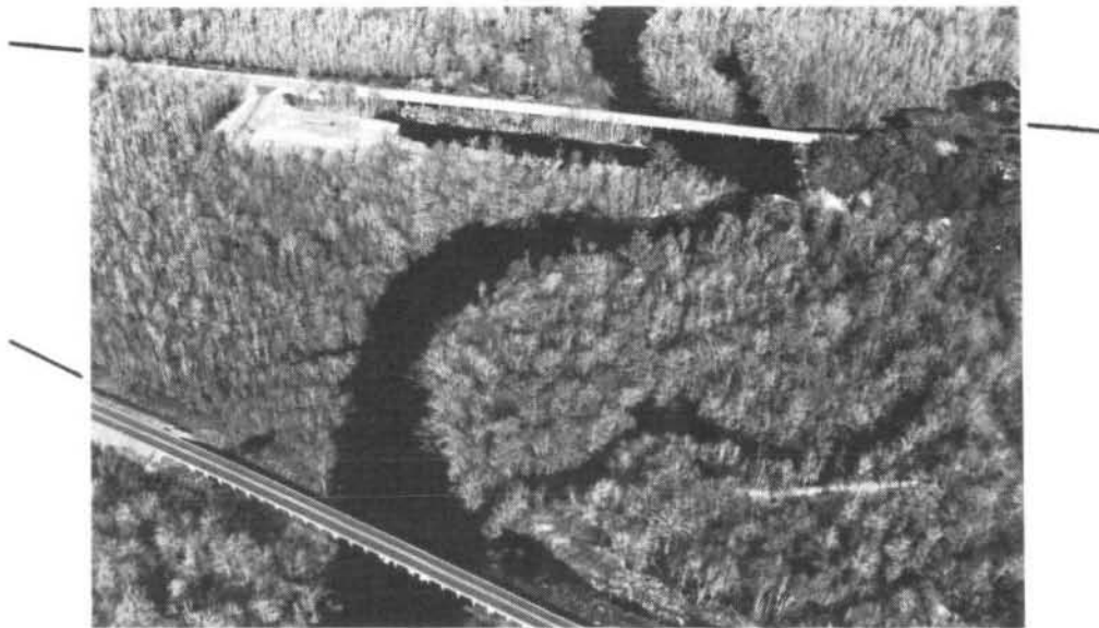
FIGURE 3 - TWO UTILITY LINES (R.M. 40.1) AND (R.M. 40.4) (WITH SEABOARD COAST LINE RAILROAD BRIDGE, FOREGROUND, AND U. S. 17A HIGHWAY BRIDGE, BACKGROUND)
