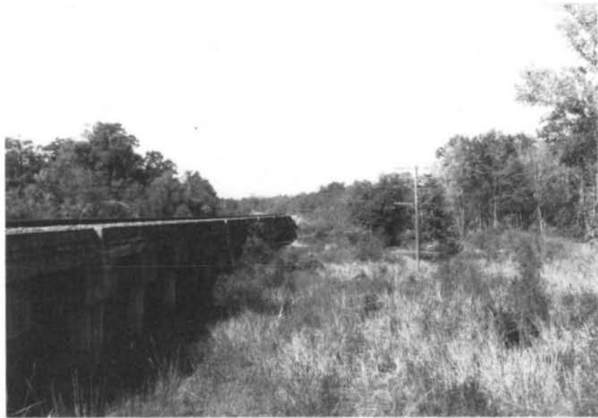
FIGURE 2 - SEABOARD COAST LINE RAILROAD BRIDGE (R.M. 40.1)
