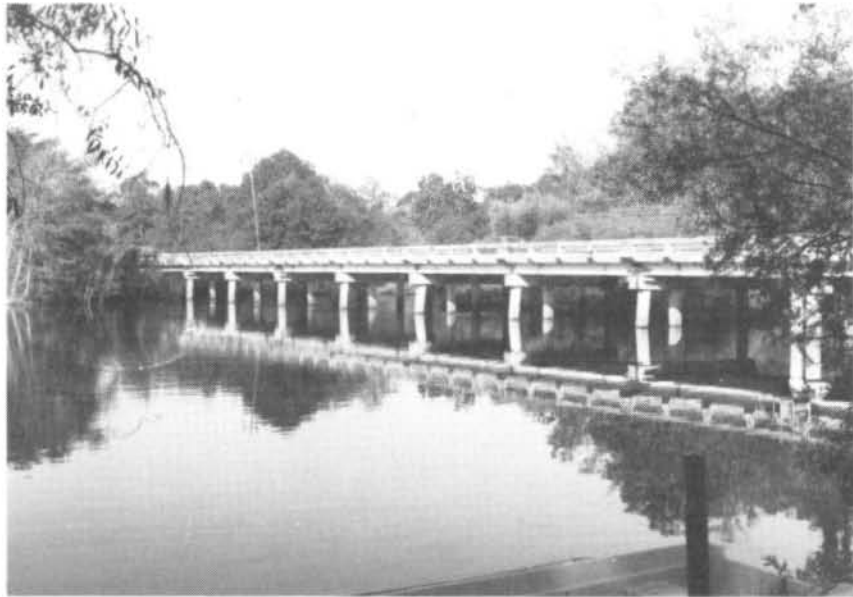
FIGURE 4 - U. S. 17A HIGHWAY BRIDGE (R.M. 40.4)
