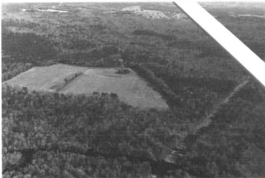
FIGURE 5 - UTILITY LINE (R.M. 41.2)
