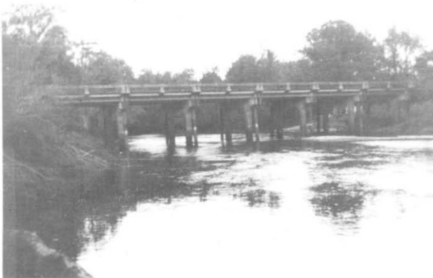
FIGURE 8 - U. S. 76 HIGHWAY BRIDGE (R.M. 59.0)
