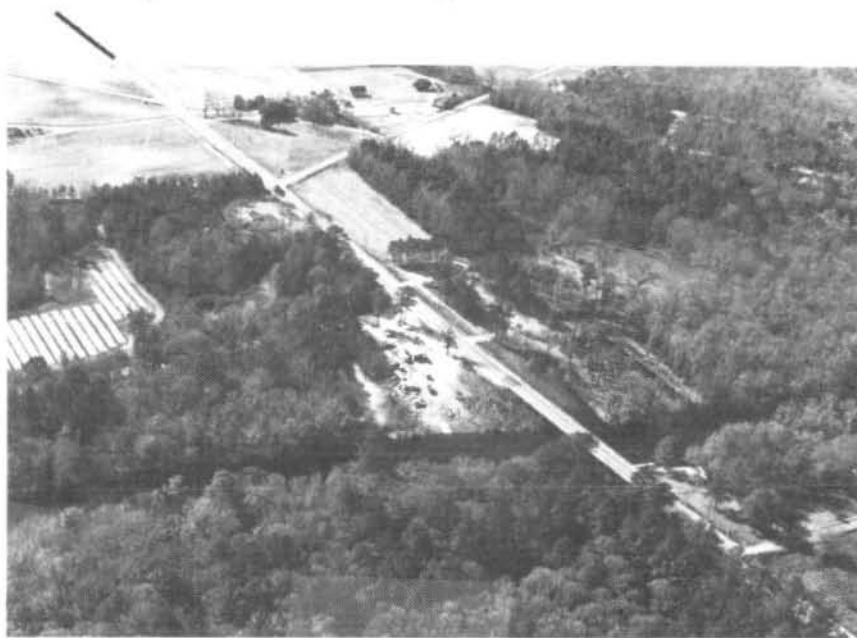
FIGURE 9 - UTILITY LINE (R.M. 59.0) (AND U. S. 76 HIGHWAY BRIDGE)
