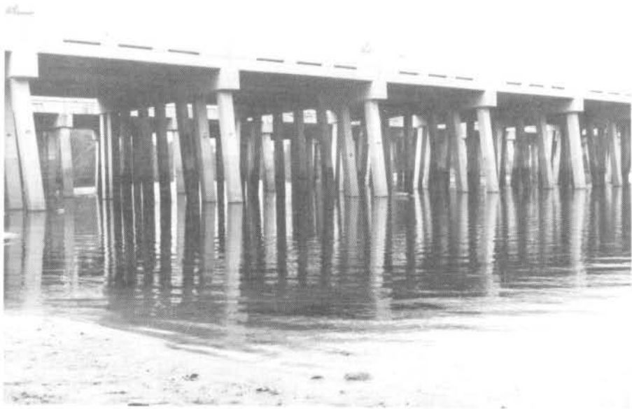
FIGURE 5 - U. S. 501 HIGHWAY BRIDGES (R.M. 41.7)
