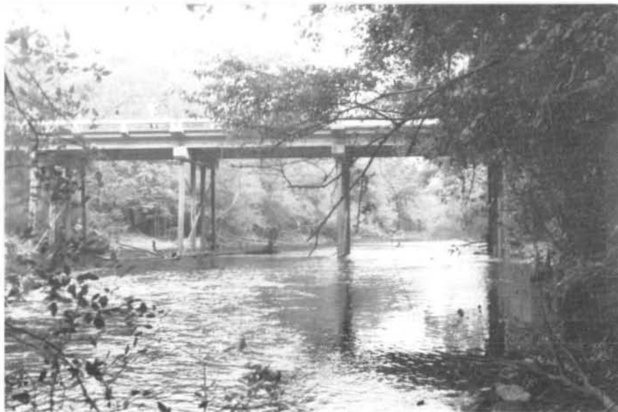
FIGURE 9 - S. C. 377 HIGHWAY BRIDGE (R.M. 78.9)
