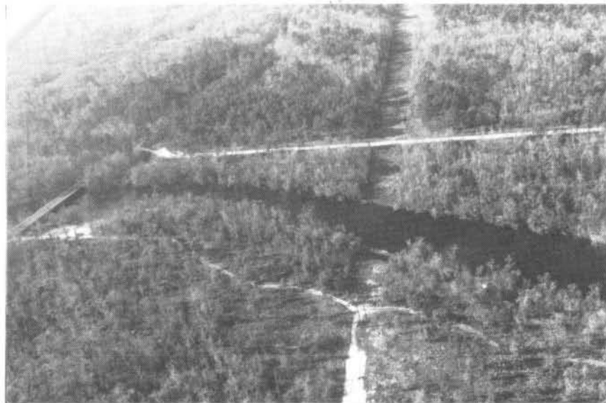
FIGURE 5 - UTILITY LINE (R.M. 68.0)
