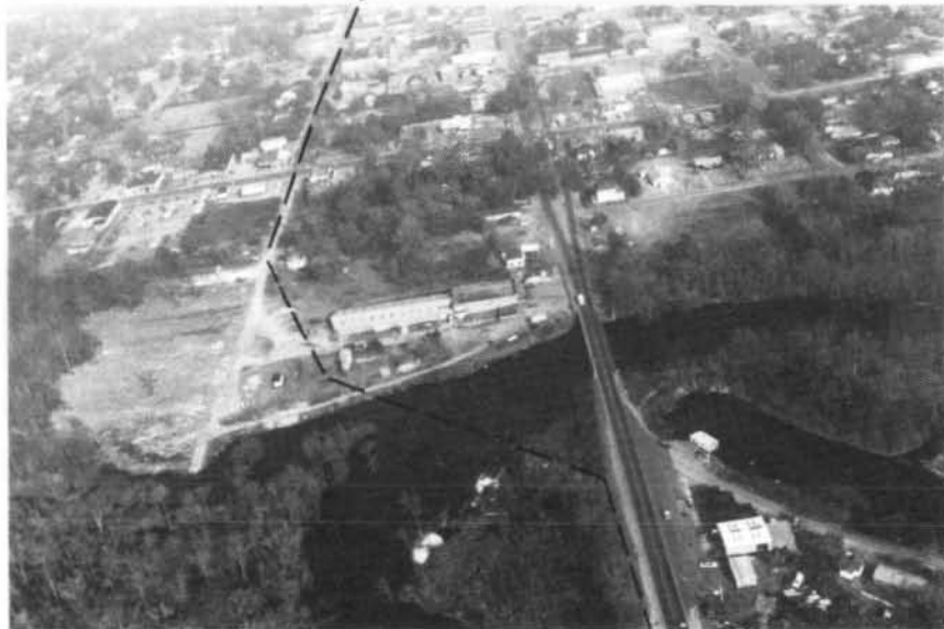
FIGURE 15 - UTILITY LINE (R.M. 86.7) (AND U. S. 52 & S. C. 261 HIGHWAY BRIDGE)
