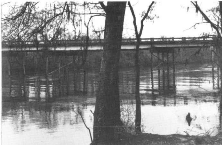
FIGURE 3 - S. C. 41 HIGHWAY BRIDGE (R.M. 48.5) (AND UTILITY LINE)
