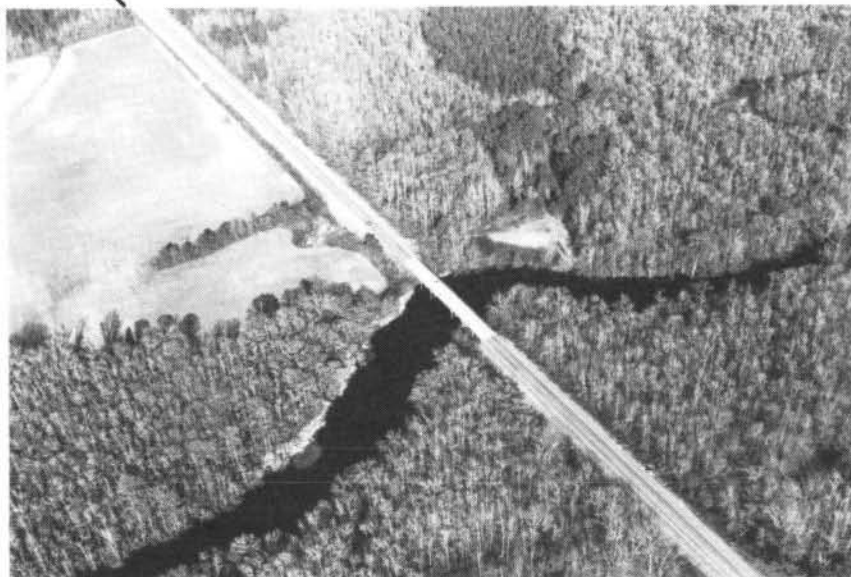
FIGURE 19 - UTILITY LINE - BLACK MINGO CREEK (R.M. 9.9) (AND S. C. 41, 51 HIGHWAY BRIDGE)
