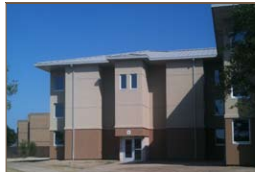
An example of an unrenovated VOLAR barrack can be seen on the left behind this newly renovated VOLAR barrack at Fort Hood. Photo by Jill Alexander
