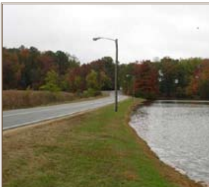
Army dams such as the Lake Eustis Dam at Joint Base Langley-Eustis, Va., which has a roadway on top are assessed for regulatory compliance during Triennial Reviews. Photo by Dwayne Smith
