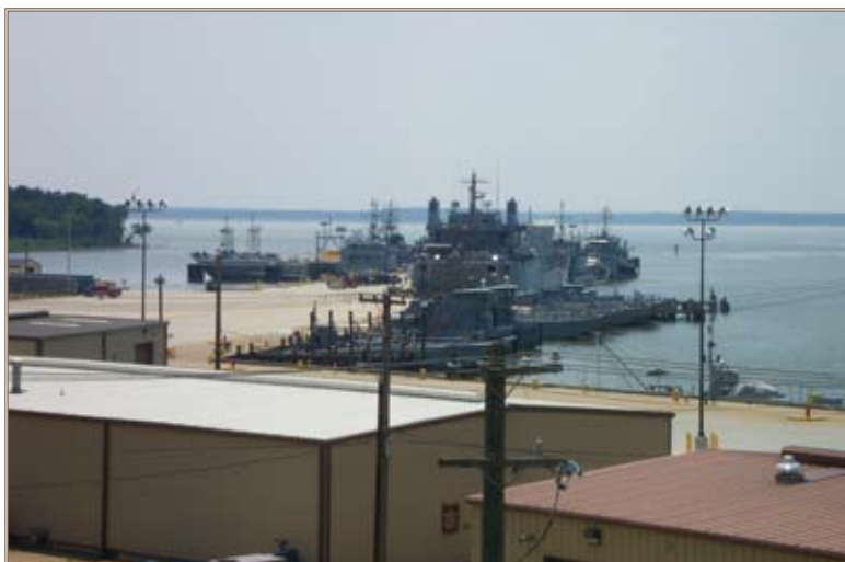
Army waterfront facilities fall under the ATIP. Photo by Mary Beth Thompson
