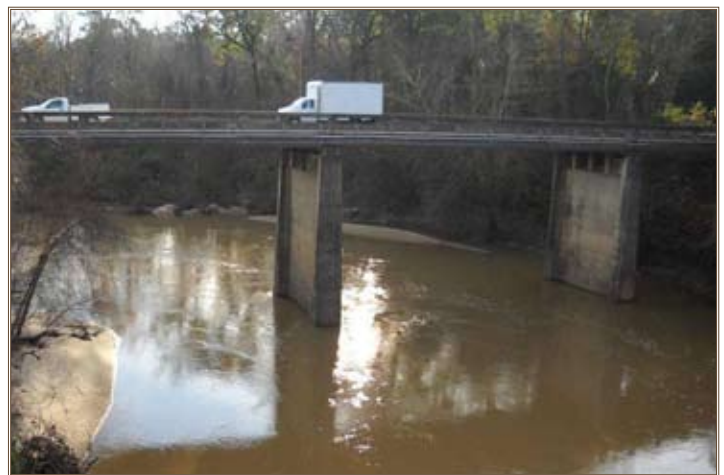
Army bridges are inspected every two years. Photo by Kenneth Renfro
