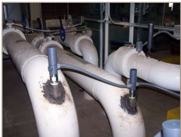
Zeta Rods are installed into grounded pipes or vessels, which serve as one electrode in the capacitor.
