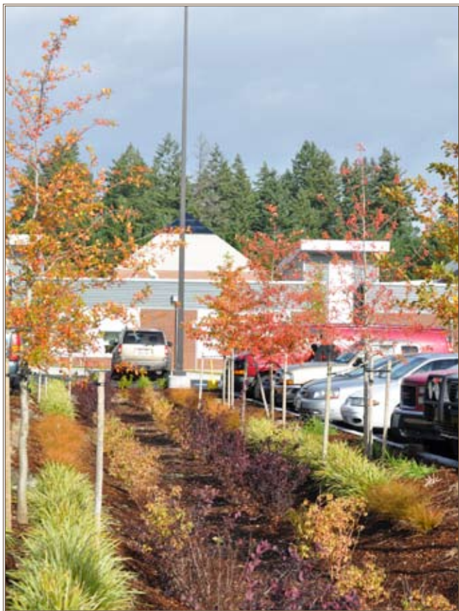
The Nisqually Medical and Fulton Dental clinics’ grounds at JBLM contain four rain gardens, which control water pollution on the site. Photo by Andrea Takash
