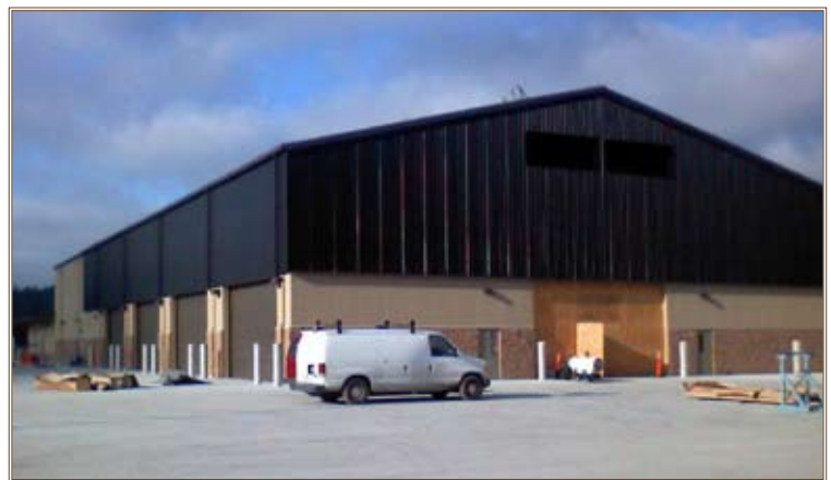
The new tactical equipment maintenance facility at JBLM features transpired solar collectors, which contribute to the building's energy efficiency. Photo courtesy of Belay Architecture
