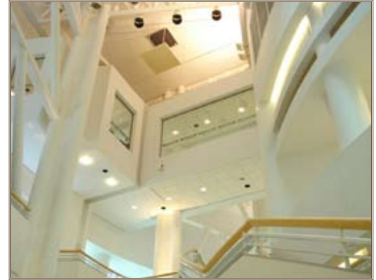
Changing lights at 90 feet in the air presents a safety challenge that the designers of the atrium at Fort Wainwright’s Bassett Army Hospital did not take into account. Courtesy photo
