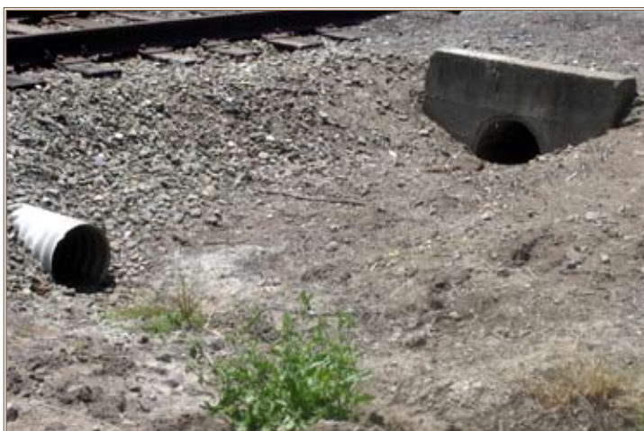
Drains and culverts are visible features that aid survey crews.
