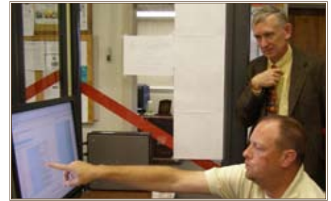
Gregory Bean (standing), Fort Bragg’s director of Public Works, and Coby Jones, UMCS manager, review the status of Fort Bragg’s building automation system at the UMCS workstation. U.S. Army photo
