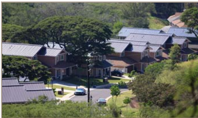
Possibly one of the most sustainable neighborhoods built on an Army installation, Fort Shafter's Simpson Wisser neighborhood is part of the U.S. Green Building Council's Leadership in Energy and Environmental Design for Neighborhood Development pilot, which will help establish the first national green ratings for neighborhood development. Photo by Mark Brown, IPC
