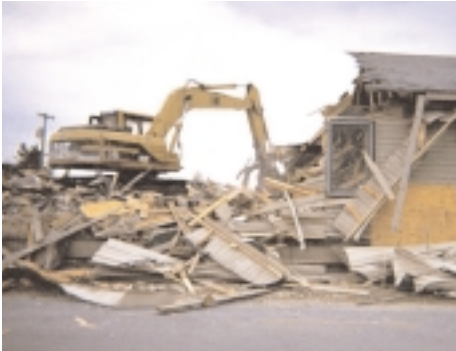
Building T-215 partially demolished.
