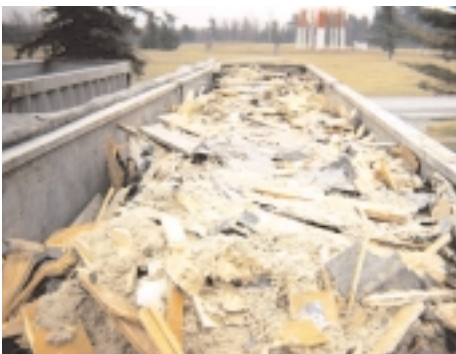
Building T-215 loaded debris material in trailer.
