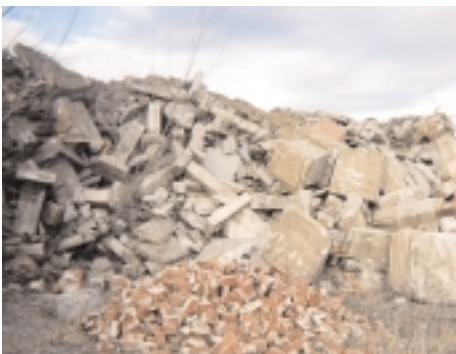
Building T-215 concrete and brick debris at reclamation site.
