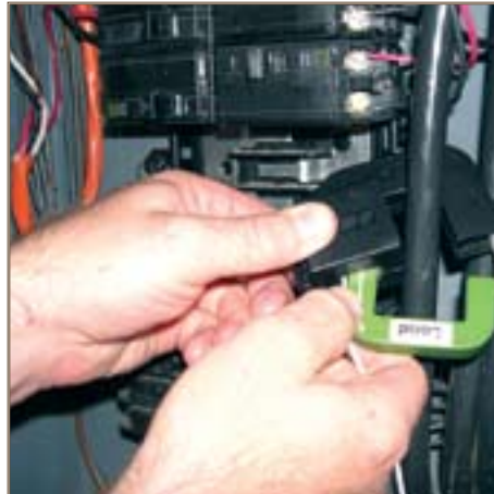
Two-volt output split-core current sensors installed noninvasively around the electrical feeds allow for a quicker, safer install that does not require the load to be shut down for installation. Photo courtesy of E-Mon LLC
