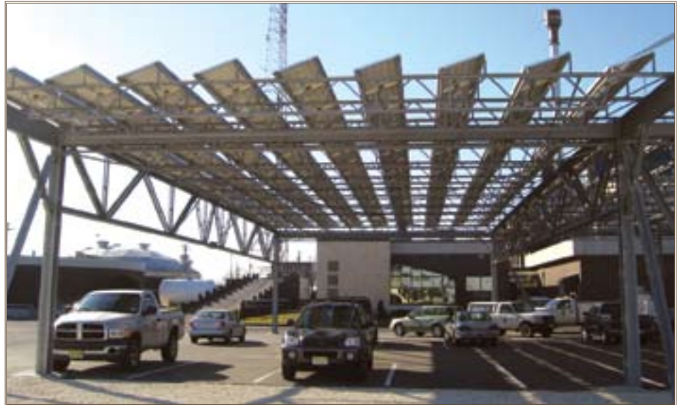
Solar power panels on a photovoltaic carport project in Atlantic City, N.J., are similar to what is being constructed by the Corps for the New Jersey National Guard. Photos by Armando Jimenez, U.S. Army Corps of Engineer, New York District
