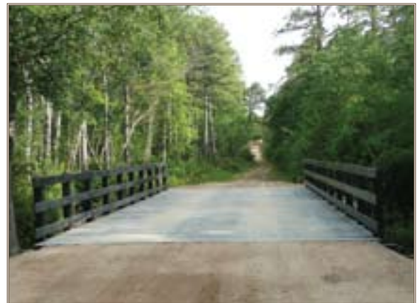
Fort Bragg’s recycled thermoplastic bridge is equipped with sensors for remote monitoring to collect performance data.
