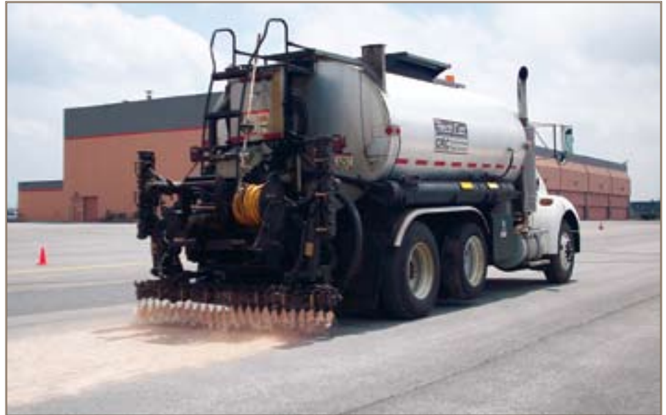
A seal coat is applied to a test strip on the airfield tarmac at Fort Drum, N.Y., as part of the Army Transportation Infrastructure Program's testing of airfield seal coats. See story on page 11. Photo courtesy of Ali Achmar
