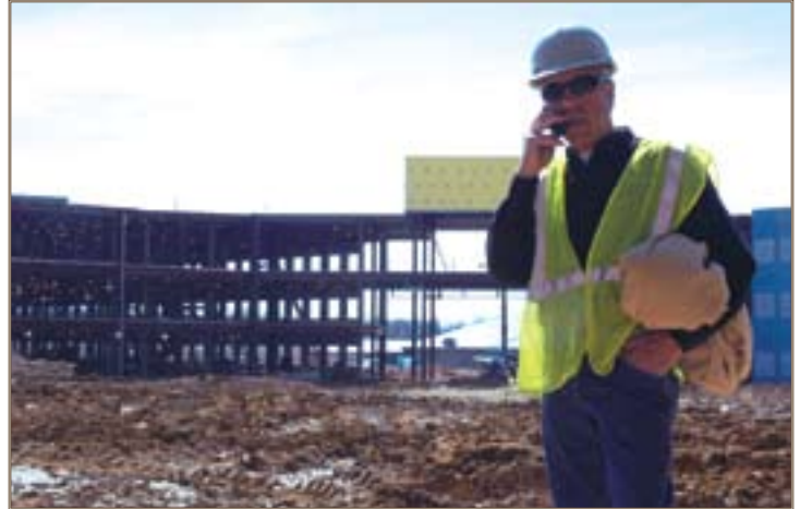
A contractor talks to his boss at the site of the Human Resources Center of Excellence.
