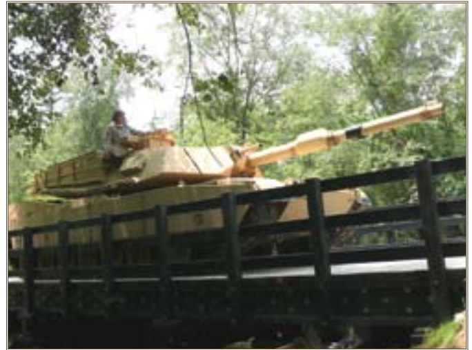
An M-1 tank crosses the new recycled thermoplastic bridge at Fort Bragg. Photos by Dr. Tom Nosker, Rutgers University
