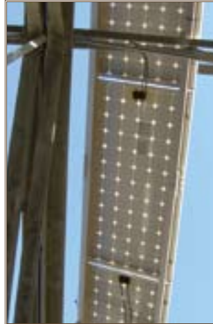
The solar power panels are composed of modules, and each module is made up of several solar photovoltaic cells that absorb the sun’s light and produce electricity.
