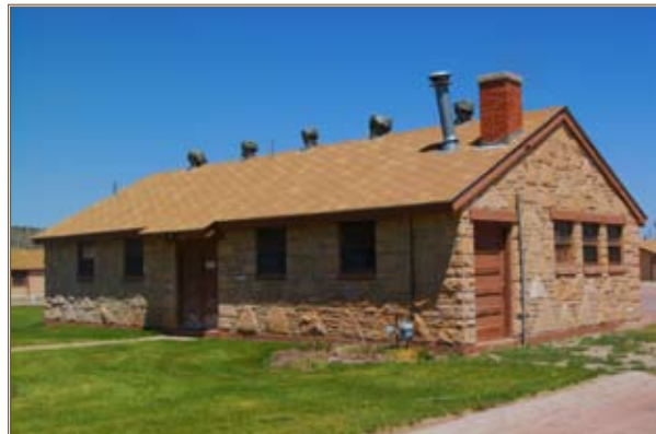
Building 301, constructed with locally quarried sandstone as a Works Progress Administration project, is an excellent example of Camp Guernsey's unique historic stonework. Photo courtesy of Mary Humstone, University of Wyoming American Studies Program
