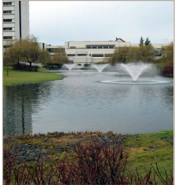
Aerator fountains in Madigan's detention pond lower the temperature of water discharged from an on-site National Priorities List site.
