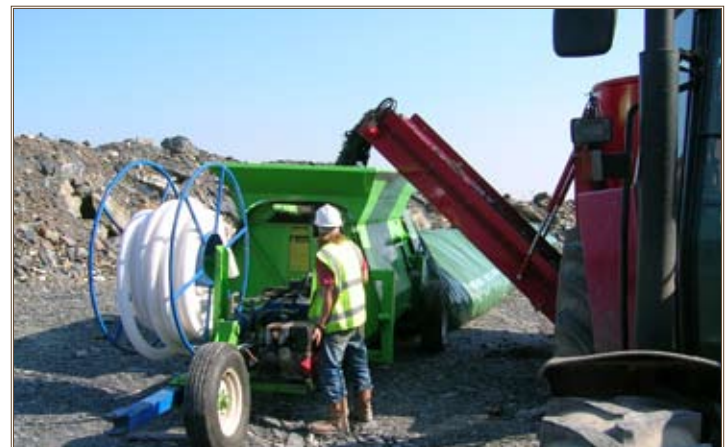
A worker oversees the placing of material into the EcoPod.
