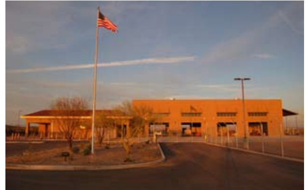
The Arizona DEMA’s new field maintenance shop is on track to become LEED Gold certified. Photo courtesy of Arizona DEMA
