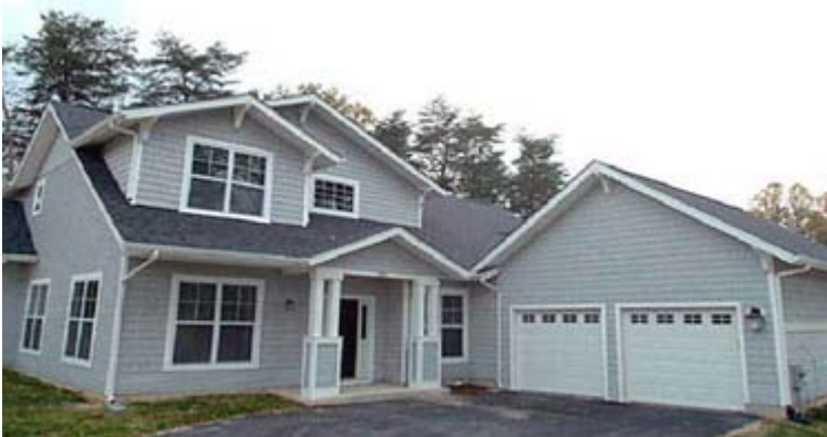
Field Grade Officer housing, complete with 2 car garages, borders the golf course at Fort Meade, Maryland.
