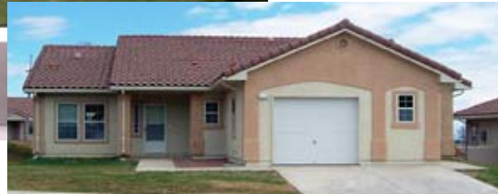
New family housing unit on Fort Huachuca built with Army Family Housing MILCON funds.
