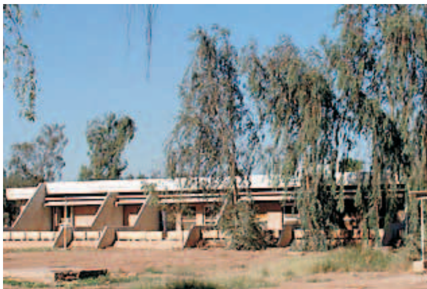
This section of the existing Iraqi air force hospital on Balad Southeast, now Logistical Staging Area Anaconda, will be renovated to serve as administrative space and medical logistical storage for a modular hospital to be built as a separate project.
