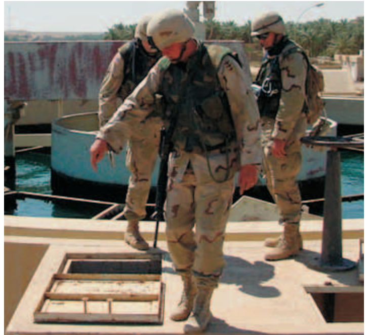
CPT Guy Joseph, 248th Combat Heavy Company attached to the 130th Engineer Brigade (front), along with CPT Edward "Ed" Chamberlayne (rear) and Fritz Ligday (right), both of the U.S. Army Corps of Engineers Europe District, inspect water coagulation tanks in Baghdad, northwest of Ar Ramadi, in the 3rd Armored Cavalry Regiment's Area of Operations.
