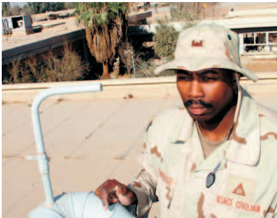
Forward Engineer Support Team project manager Hunter Dandridge looks at a ventilation system cover on the roof of the wing of a former Iraqi air force hospital to be renovated. Behind are bomb-damaged wings which will be razed to make room for a modular hospital to serve troops on Logistical Staging Area Anaconda.
