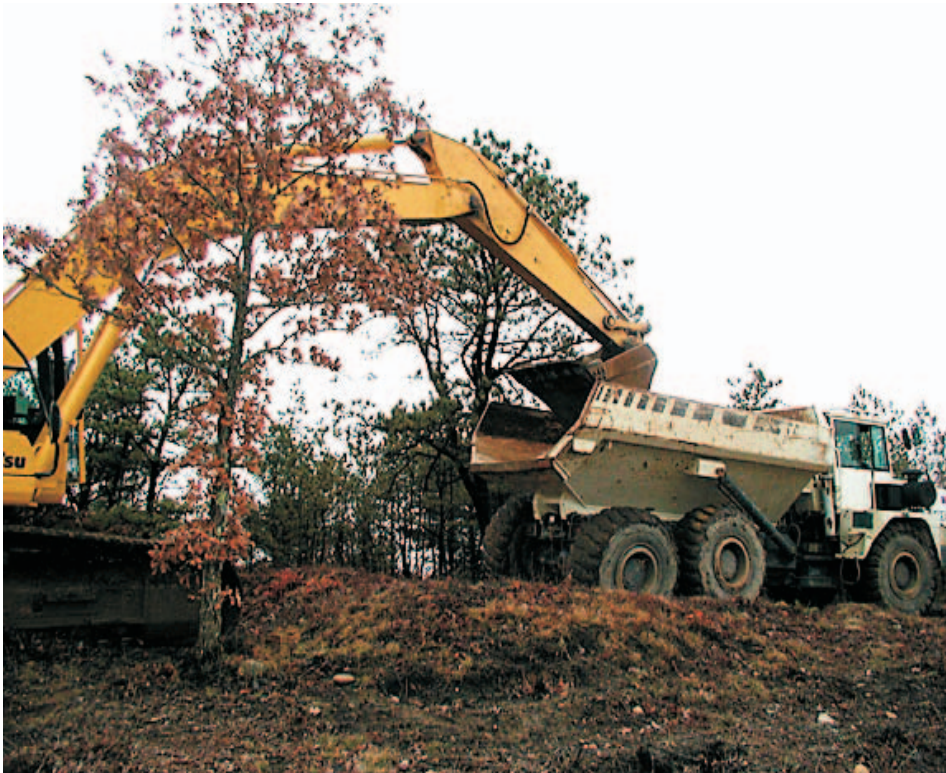
An excavator begins soil removal at Camp Edwards, Massachusetts.
