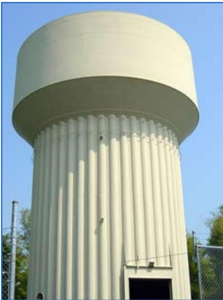
This Fort Drum water tower underwent installation of an ice free cathodic protection system to prevent corrosion even when surface ice forms in the water. Photo by Vicki Van Blaricum
