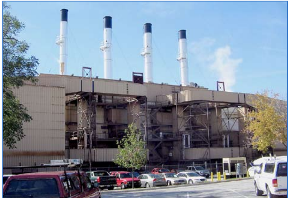
The central heating plant at Rock Island Arsenal, Ill., is shut down this summer to improve the reliability of chiller plants, create energy savings and reduce emissions of pollutants. Photo Courtesy of U.S. Army Garrison Rock Island Arsenal
