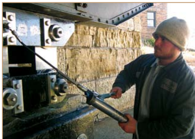
Luke Jackson, Government Bridge operator, lubricates the swing lift mechanism. Each mechanical part of the Government Bridge gets lubricated weekly. Photo by Valerie Buckingham
