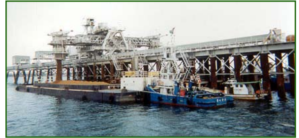
Soil from Mount Atago is loaded onto barges for transport to the land reclamation site for the new airfield at Iwakuni, Japan. Photo courtesy of U.S. Army Corps of Engineers, Omaha District
