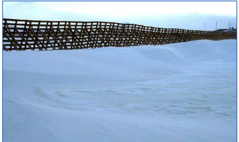
The snow fencing sculpts blowing snow into snow banks behind the fence for storage or removal. During the 2005-06 snow season, the fences saved more than $600,000 over the previous winter. Photo by Michael Sisneros
