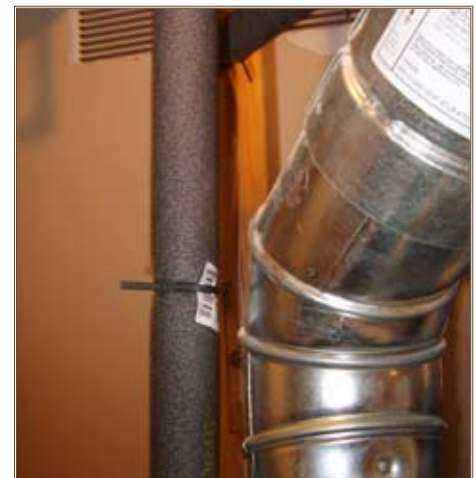
Insulated hot-water pipes deliver water that is hotter than uninsulated pipes can deliver.
