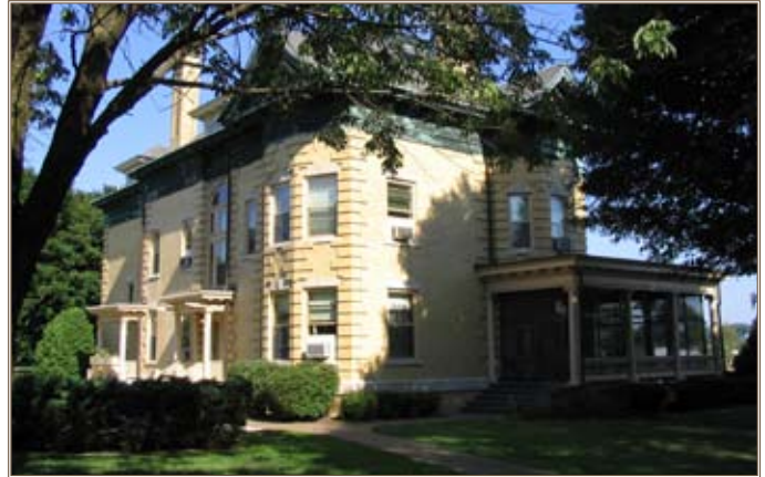
GFOQs like this one at Rock Island Arsenal, Ill., require detailed planning and upkeep. Photo courtesy of Directorate of Public Works, Northeast Region, Installation Management Command
