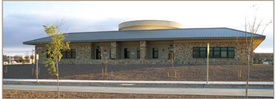
A tiger team is addressing Fort Bliss's increasing electricity and water needs from new facilities being constructed to meet growth, like this dining facility. Photo by Donald Vincent, Fort Bliss Department of Public Works' Energy Office
