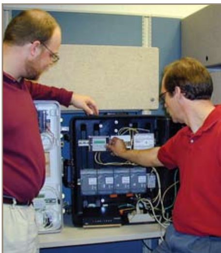
Joe Bush (left) and David Schwenk of the Construction Engineering Research Laboratory work on a direct digital control panel. By implementing open standards for building automation systems, components such as direct digital controls will no longer be limited to a single vendor's product line. Photo by Dana Finney
