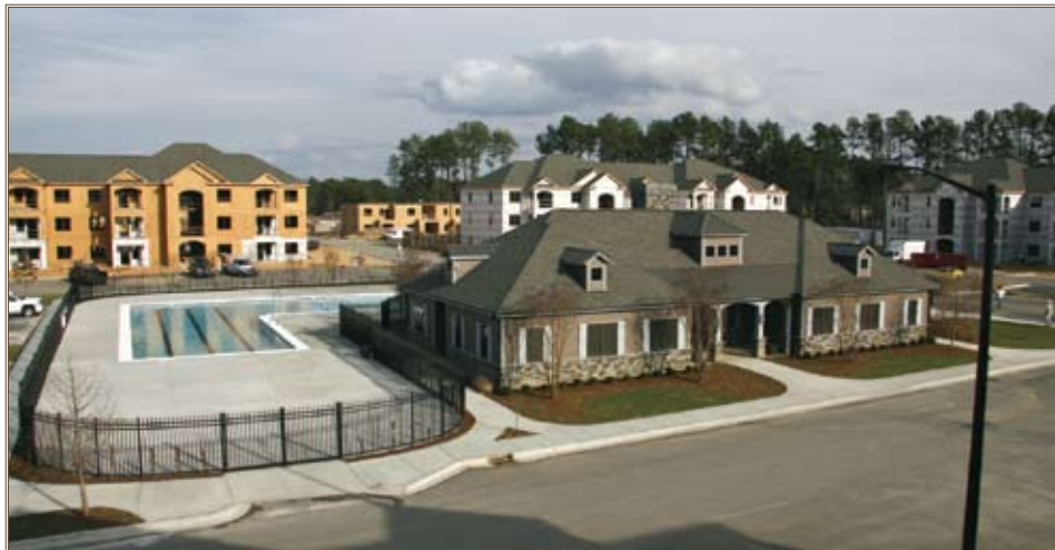
The Randolph Pointe Clubhouse and pool are centrally located at Fort Bragg's new community for senior single or unaccompanied Soldiers and surrounded by 13 three-story apartment buildings. Photos by Scarlett Tyner
