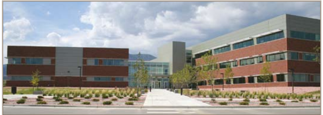
The Fort Carson 1 BCT and Battalion Headquarters received a LEED Gold for New Construction certification, the Army’s first. Photo by Susan C. Galentine
