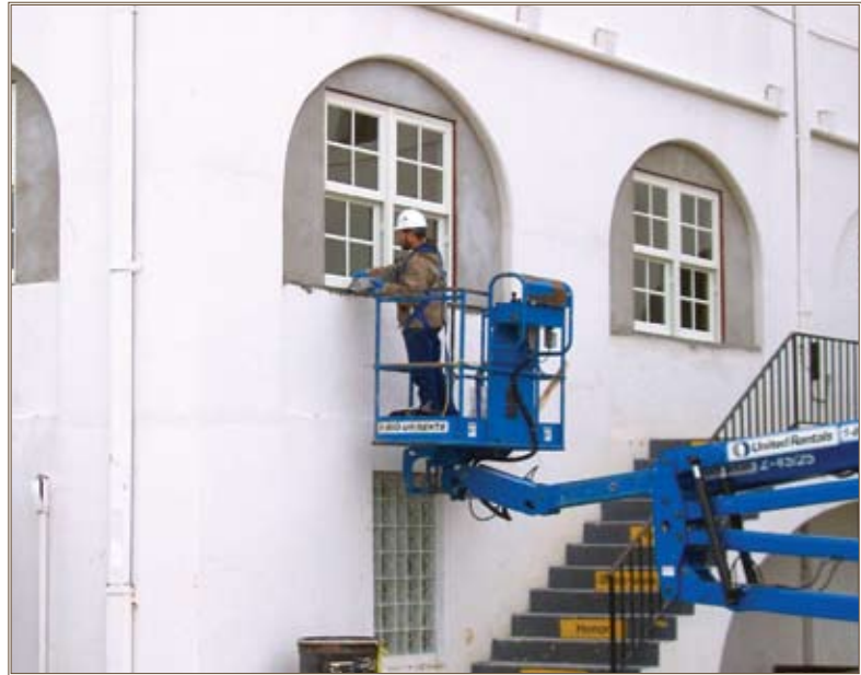
A construction worker completes window renovations on Building 2791.
