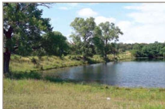
Army dams, like the Heiner Lake Dam at Fort Hood, Texas, are inspected according to FEMA guidance.
