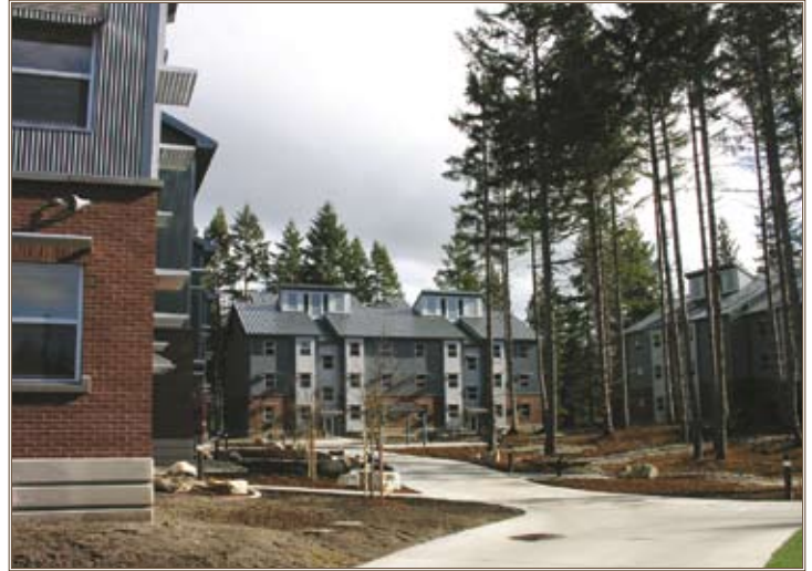
The FY 2006 Barracks complex, a Chief of Engineers Design and Environmental Honor Award winner, was designed to preserve the surrounding trees, built with exterior sunshades and oriented to maximize daylighting. Photos by Jeanette Fiess
