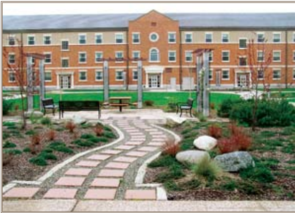
This FY 2003 Barracks courtyard features native landscaping and pavers set in pea gravel to allow storm water run-off.
