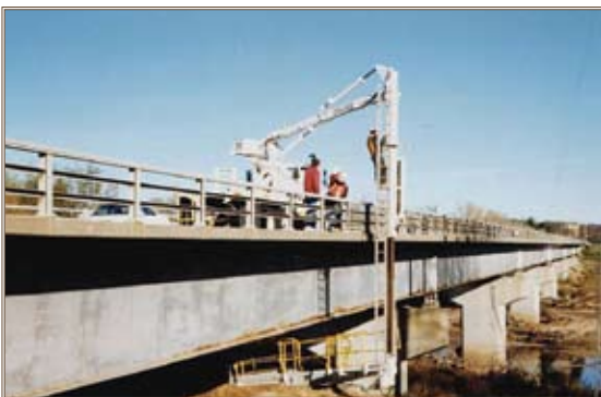
A bridge at Fort Riley, Kan., undergoes its biannual safety inspection.
