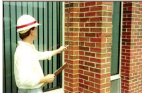
BUILDER uses a combination of inspection and condition indexes to manage building maintenance and repair. Photo courtesy of ERDC
