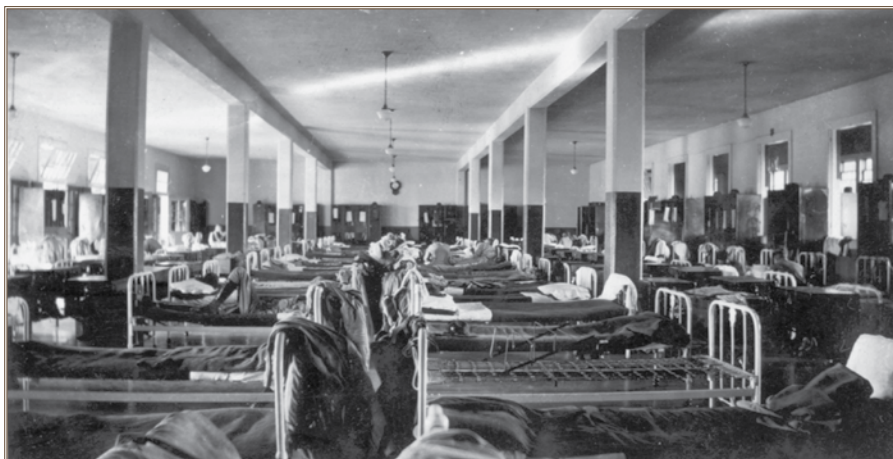
Where open-bay sleeping quarters like these were once the norm, Soldiers' living accommodations are getting an overhaul at Schofield's quads. U.S. Army photo
