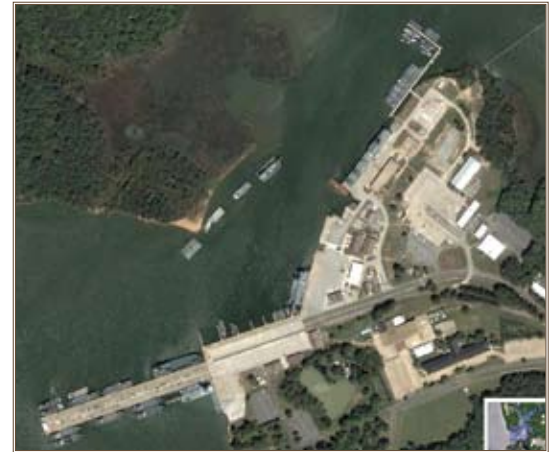
Guidance is being established for inspection of the Army's ports, like this one at Fort Eustis, Va., and other waterfront facilities.
