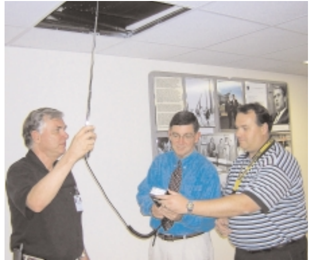
(Left to right) Bob Quick, Resource Efficiency Manager, William (Bill) Porr, Director, Directorate of Public Works, and Mark Smith, Energy Manager, Directorate of Public Works, monitor air velocity in an air plenum.
