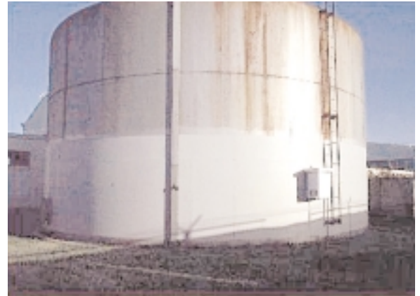
Patch test of overcoating on deluge tank.
