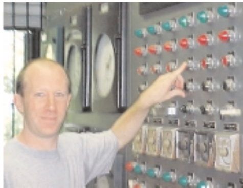
Chris Campbell, Certified Water Plant Operator, operates water pump from a remote site.
