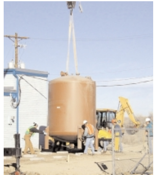
Installing the water treatment system for the city of Avondale.
