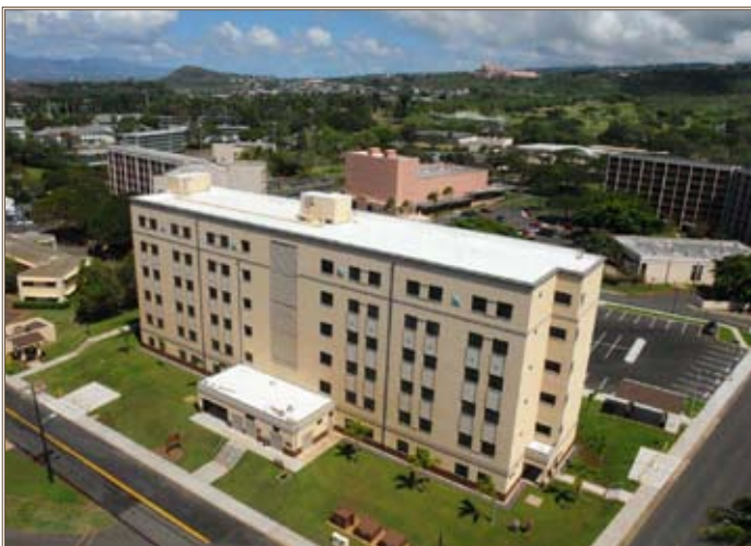
The new six-story Fort Shafter barracks houses 156 Soldiers and consumes 30 percent less energy than older barracks in use today. Photo courtesy of U.S. Army Hawaii
