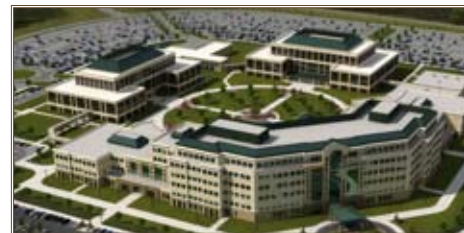
This rendering depicts how the Von Braun Complex at Redstone Arsenal will look when completed. Graphic by LS3P Associates Ltd
