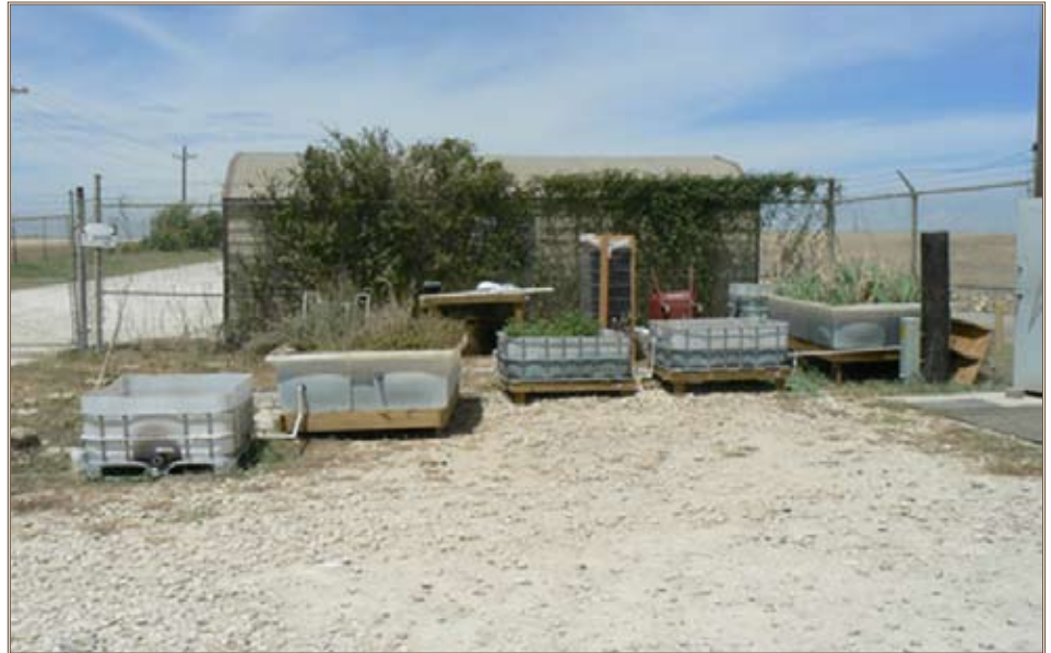
A novel microbial mat and polishing system did not meet pilot test goals for treating leachate from Fort Hood's landfill. Photos courtesy of Engineer Research and Development Center
