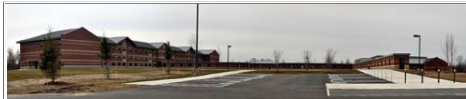
The Fort Drum WIT Complex comprises a company operations facility and a 144-Soldier barracks. Photo by Chris Gardner
