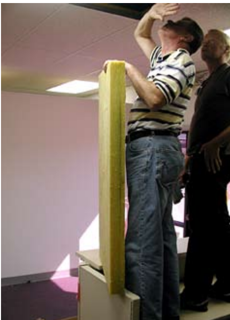
Engineers check ceiling and roof insulation to determine adequacy.
