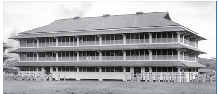
This historic barracks exhibits inherent energy-conserving features, such as a crawlspace, screened windows, deep overhangs, ridge ventilators and hip-on-gable vents. Photo courtesy of Engineer Research and Development Center
