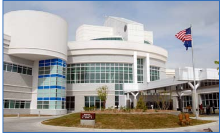
In a heat loss study, a "visual image," like this one of the new Bassett Army Hospital, is used for comparison to an infrared image like the one below. Photo by Tom Findtner, U.S. Army Corps of Engineers, Alaska District.
