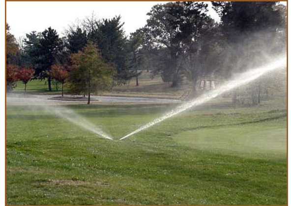
Sprinklers at the Fort Meade, Md., golf complex use nonpotable reclaimed water from wastewater treatment to irrigate. Photo by Christine Frankovitch
