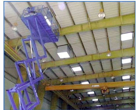
New daylighting retrofits for Army facilities in Hawaii include new skylights in a bangar at Wheeler Army Airfield. Photo by Scott Bly
