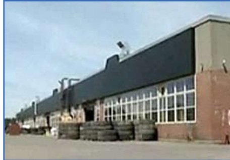
Solar walls, like this one at Fort Lewis, Wash., reduce the heating of buildings. Photo by Jini Ryan
