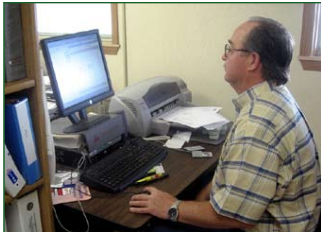
Dick Strohl, Fort Hood Directorate of Public Works engineering technician, logs into the LON Works system to monitor, control and manage the installation's systems. Photo by Christine Luciano
