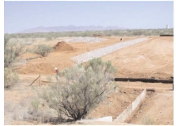
The City of Sierra Vista and Fort Huachuca have been working cooperatively on recharge basin projects to help capture precipitation runoff to recharge the Upper San Pedro Watershed for protection of the San Pedro River (photo by John Roberts)
