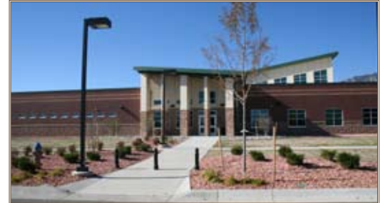
Fort Carson's new band facility realized enough project points to pursue LEED Gold certification. Photos by Susan C. Galentine
