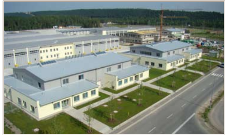
Four of the 28 company operation buildings (two per structure), with their accompanying vehicle maintenance shops behind, are completed and in use at Grafenwoehr. Beyond them, another four company operations buildings and vehicle maintenance shops are under construction. Photos by Andrea Hoesl, Directorate of Public Works, Grafenwoehr
