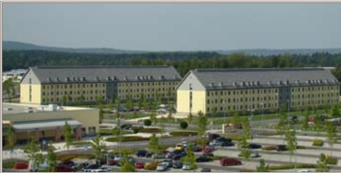
Two of the 12 new barracks buildings near completion at Grafenwoehr.
