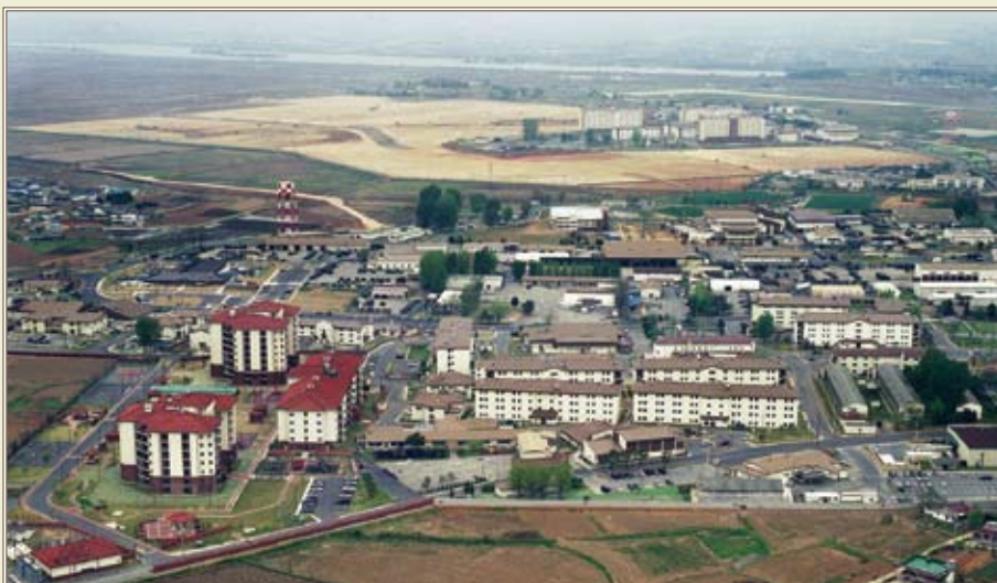
Construction is ongoing on the newest land at USAG Humphreys, called Parcel One (top of photo). When the transformation of Humphreys is complete, the installation will almost triple in size and be home to nearly 45,000 people.
