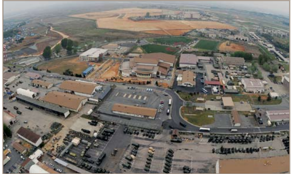
The old and the new share space at USAG Humphreys, South Korea. Here, construction is underway on the newest land, dubbed Parcel One (top of photo). Photos by Bob McElroy
