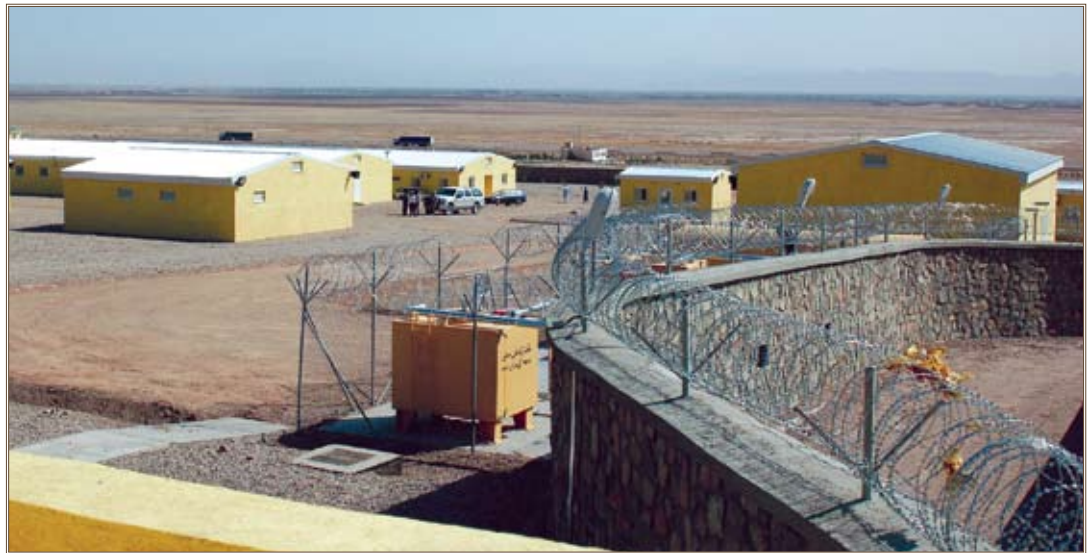
This base shows typical ANA base new construction.
