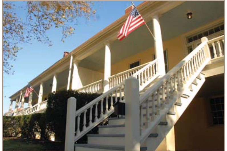
The Rookery on Fort Leavenworth, Kan., has undergone updating and restoration. Photos by Prudence Siebert, Fort Leavenworth Lamp
