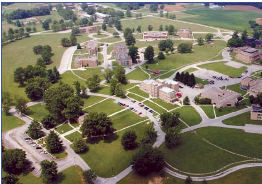
This aerial photograph shows some of the 980-acre property that the Indiana National Guard acquired and converted into the Muscatatuck Urban Training Center. Photo courtesy of Karstin Carmany-George
