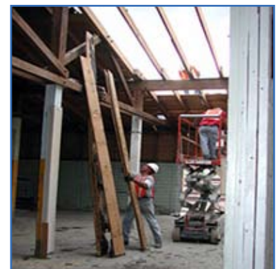
Workers deconstruct a World War II-era warehouse at Fort Carson, Colo.
