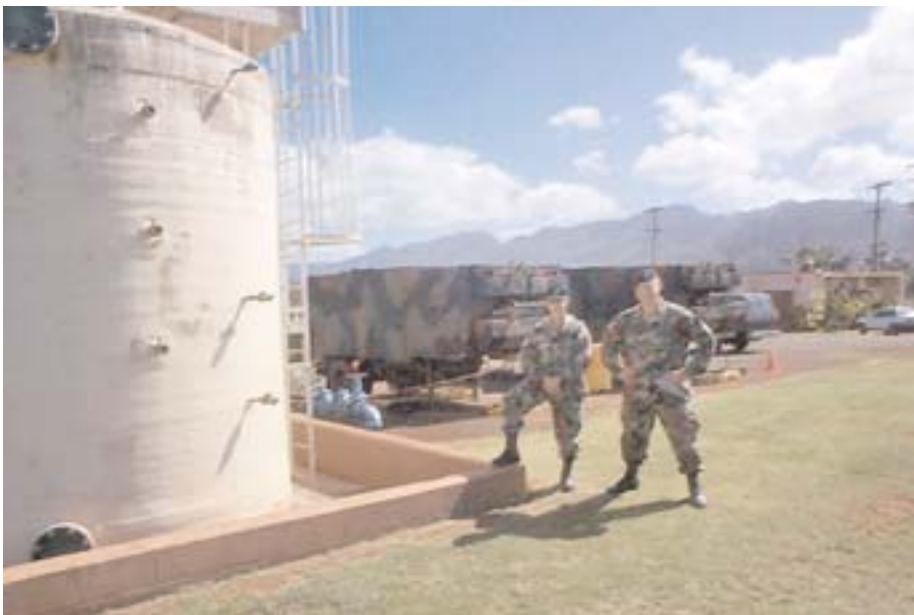
CW3 Patti Shoefstall, and the author pose in front of two of the Army's new Deployable Power Generation and Distribution Systems (DPGDS) currently providing backup power to the wastewater treatment plant.
