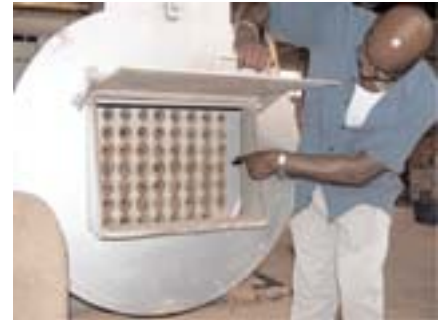
Army Energy Awareness Program Manager, David Williams inspects a fire-tube boiler at the Fort Bliss Headquarters building.
