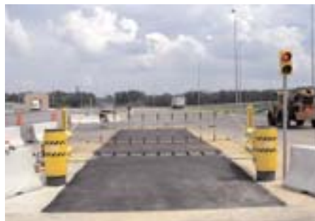
The ground-retractable automobile carrier (GRAB) at Fort Hood.
