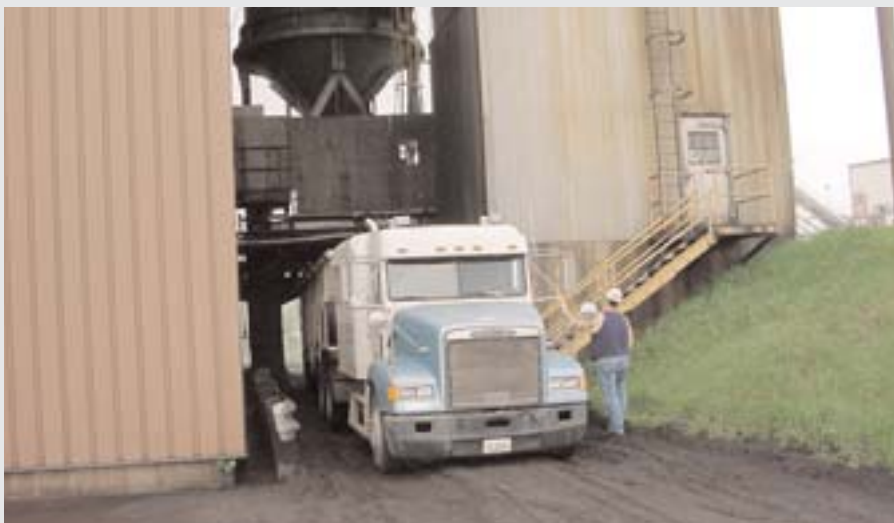
American Ordnance employee, Jerry Burnett, oversees loading 22 tons of fly ash into a semi for transport to a cement company for recycling. Recycling the fly ash from the Iowa Army Ammunition Plant's coal-fired heating plant saves landfill space.
