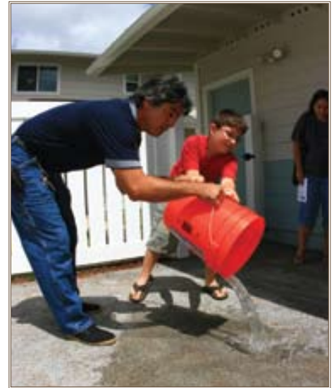
Schofield Barracks Family Housing resident William Brown gets some help from AHFH maintenance technician Baron Loftin to demonstrate how quickly permeable concrete — one of the many LEED Gold features — absorbs water. Photo courtesy of AHFH
