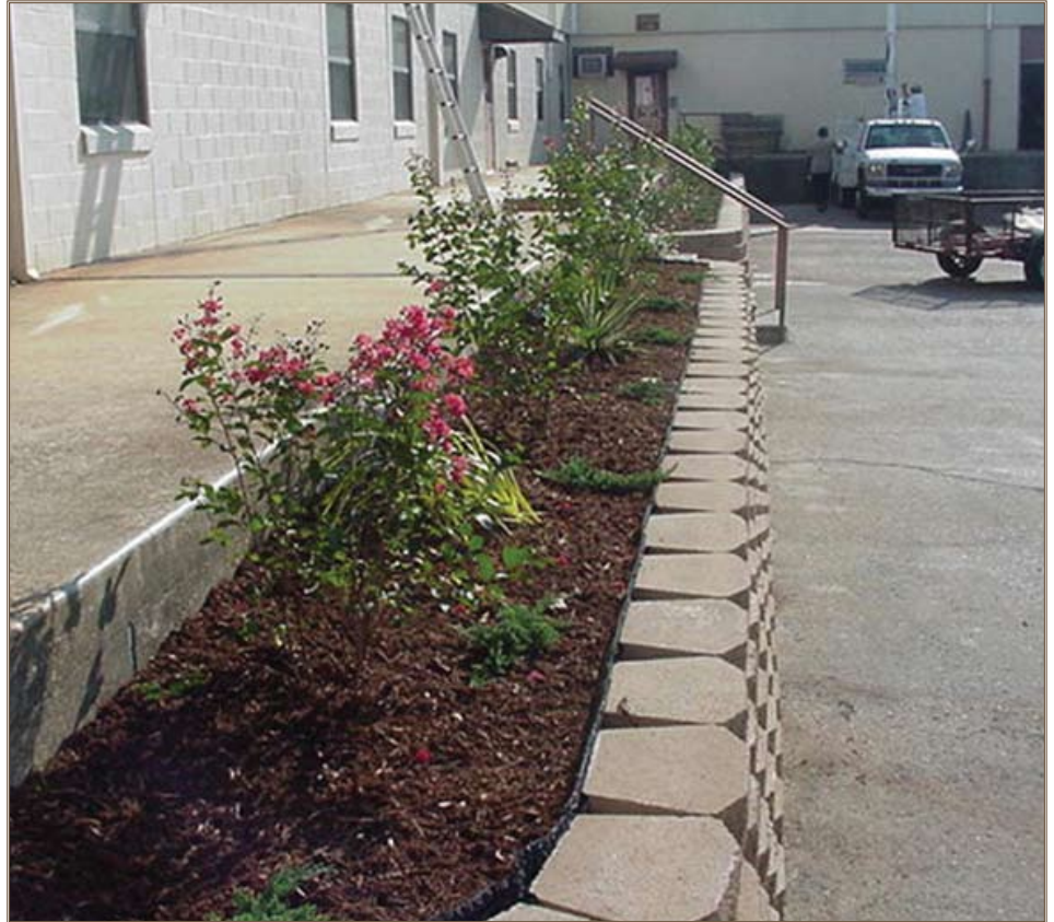
Channeling rainwater runoff to beneficial uses, such as bioretention for landscaping, is one way to recycle. Photo courtesy of U.S. Army Corps of Engineers
