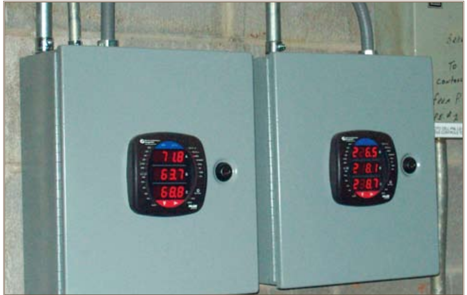
These advanced meters capture the electric use and natural gas consumption for the Redstone Arsenal (Ala.) Post Exchange and report the data to the energy manager in the Directorate of Public Works. Photo by Patrick Holmes, Johnson Controls Huntsville
