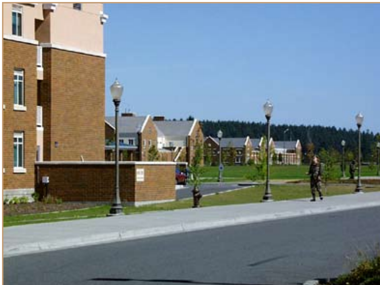
This barracks complex at Fort Lewis, Wash., is an example of the focus on quality in Soldier housing. Photo courtesy of the Office of the Chief of Staff for Installation Management
