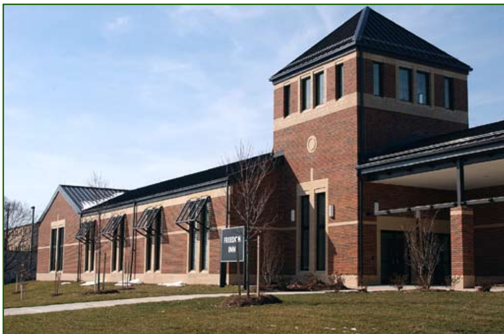
The design and construction of the 21,000-square-foot, $10-million dining facility at Fort Meade, Md., represents a tremendous step forward in military construction, offering Soldiers and civilians buffet-style dining in five dining areas, including a veranda. Photo by Travis Edwards, Fort Meade Public Affairs Office
