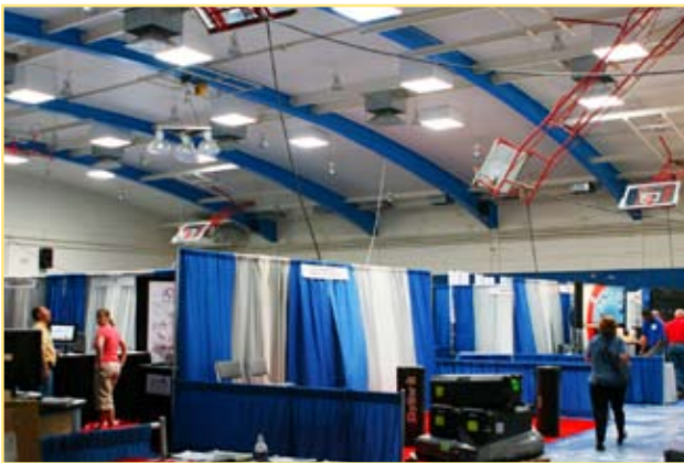
Daylighting in Barnes Field House at Fort Huachuca conserves energy by reducing the need for artificial light. Photo courtesy of Bill Stein
