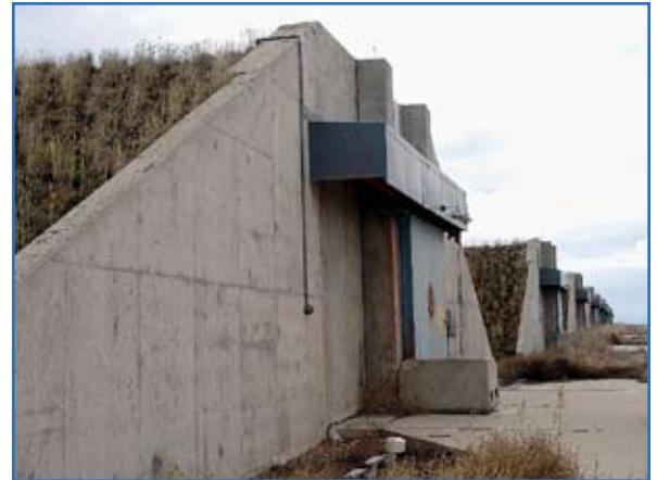
More than 20,000 World War II- and Cold War-era Army ammunition storage facilities — like this one at Tooele Army Depot, Utah — are a major compliance responsibility. Photo courtesy of U.S. Army Chemical Materials Agency
