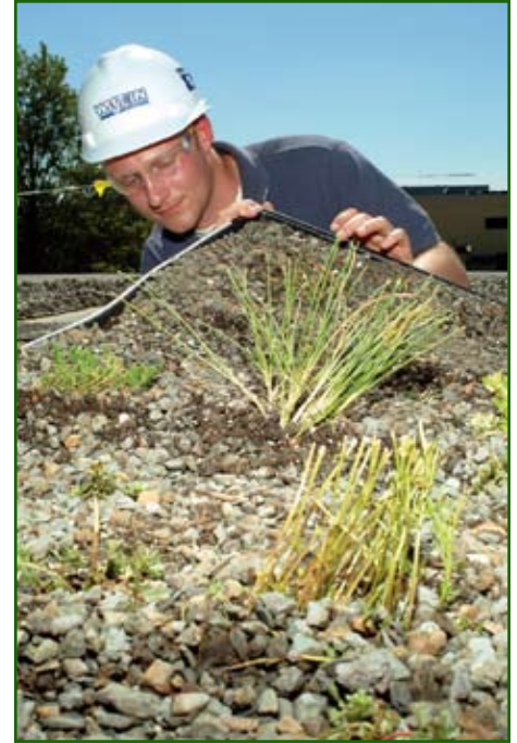
As the sedum plants grow, they will spread out and cover the entire module. The plants are drought resistant, flood resistant and able to stand up to high winds. Photo by Steve Grzedzinski
