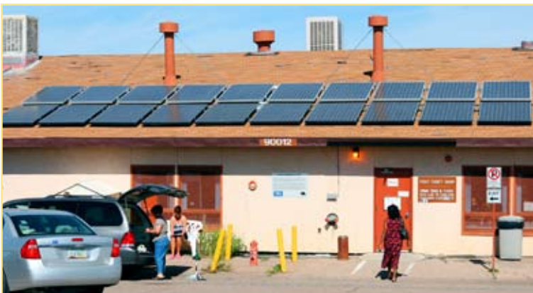
Photovoltaic panels on its roof provide a source of renewable energy for the Fort Huachuca Thrift Shop. Photo courtesy of Bill Stein
