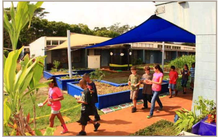
Modified downspouts deliver rainwater to 3,000-gallon rainwater harvesting tank (back center) in the Fort Shafter Elementary School’s outdoor classroom garden. Photo by Mark I. Brown, Lend Lease
