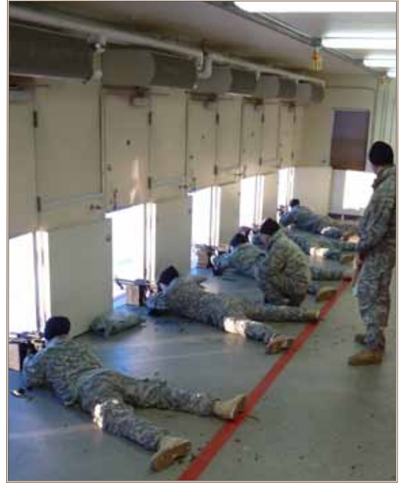
A Fort Wainwright air curtain firing range facility, demonstrated with ITTP funding, enables Soldiers to complete live-fire training in subzero temperatures. Photo by James Buska, ERDC
