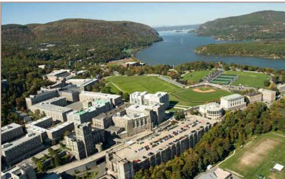
By combining ESPC with SRM funding, West Point maximizes facility infrastructure improvements and meets energy reduction goals. West Point photo
