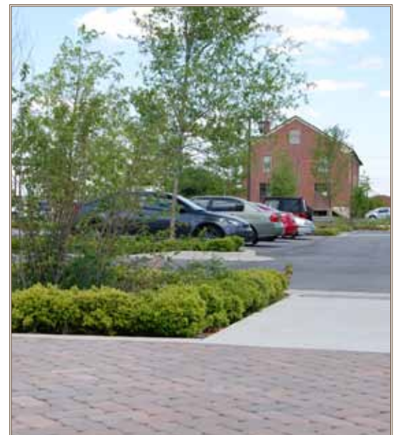
A Fort Bragg parking lot features LID water management techniques — permeable pavers, infiltration channels and rain gardens — designed to mimic the site’s predevelopment hydrology by allowing infiltration to the aquifer. Photo by Jonelle Kimbrough
