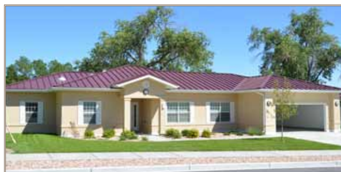
This single-family four-bedroom unit is part of the project that earned LEED Platinum at Dugway Proving Ground.
