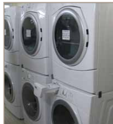
Energy Star front-loading washers and dryers use less water and energy, and can be stacked to save space. Photo by Master Sgt. Mitch Jackson
