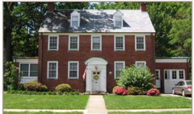
After renovation, the Colonial Revival homes in Belvoir Village feature improved kitchens where the garages used to be.
