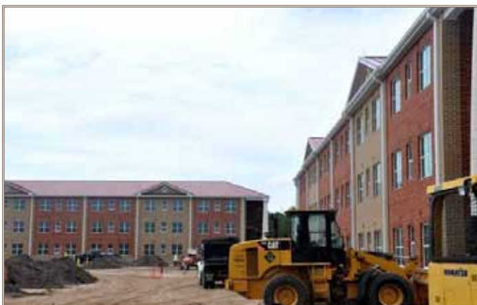
At Fort Stewart, Ga., permanent party barracks are under construction.
