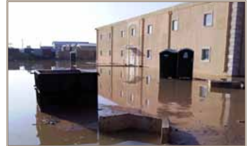
Flooding at Kandahar Air Field results from a lack of master planning and attention to drainage. Photo by Col. Stewart Fearon
