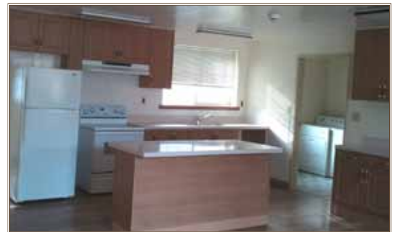
A finished Yongsan renovation product features new utilities, wallboard, fixtures and cabinets.
