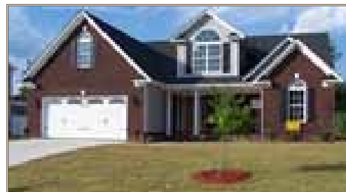
For off-post housing to be considered adequate, it must meet OSD standards of affordability, location, features and physical condition. Photo courtesy of Sandy Randolph
