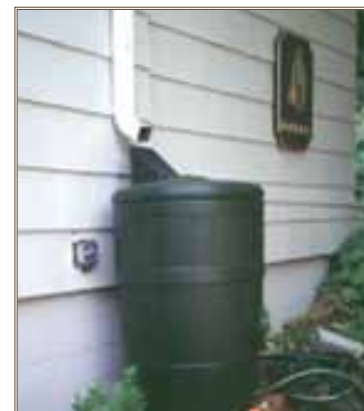
A barrel for capturing rainwater is another LID technique. Photo courtesy of Low Impact Development Center Inc.
