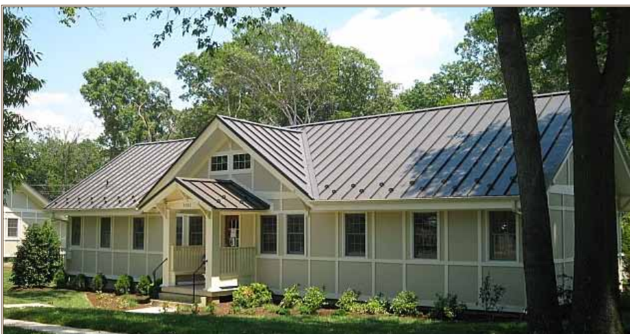
The exteriors of Jadwin Loop's six Craftsman style houses, built from prefabricated kits in the 1920s, are restored to their original character.
