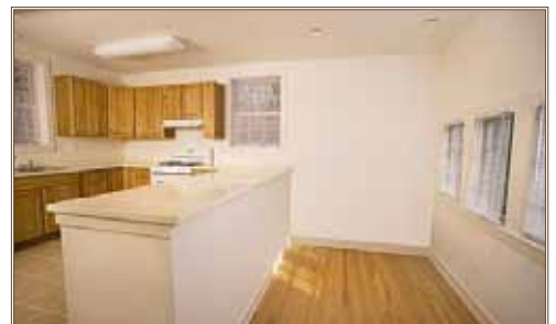
The new kitchen and dining areas of Belvoir Village homes occupy the former garage space.
