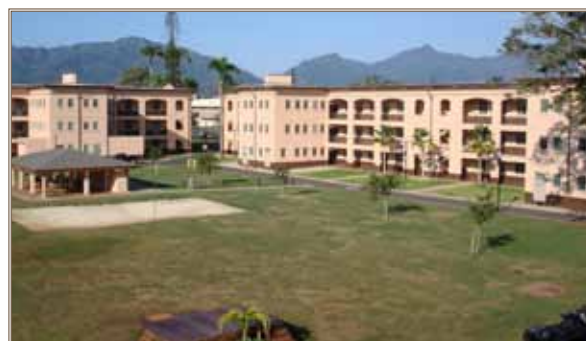
The renovated historic Quad C Barracks Complex on Schofield Barracks depicts the stunning results that can be achieved through building reuse. Photo by Ken Hayes, historic preservation specialist
