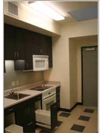
In the shared kitchen, upgraded appliances and surfaces provide ease of cleaning, and the microwave placed above the range adds counter space. Photo by Doug Symes, Portland District, USACE
