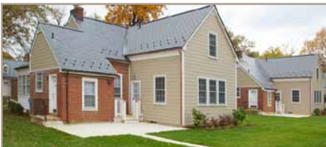
Two-story additions to the backs of Fort Belvoir's Gerber Village homes provide the homes with a modern layout and were designed with siding, roofing and windows that make the additions blend with the original design.
