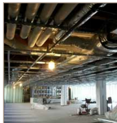
Fort Benning, Ga., Starship barracks undergo renovations inside and out.
