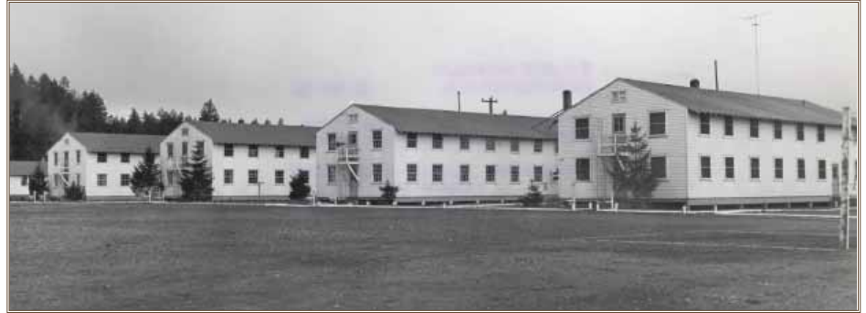
World War II wood buildings cover Lewis North in 1941. Photo courtesy of DPW Cultural Resources Section, JB Lewis McChord
