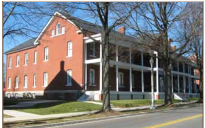
Completed Renovation of Quarter 249, built in 1909. Photo by Kristie Lalire, 10Dec12.
