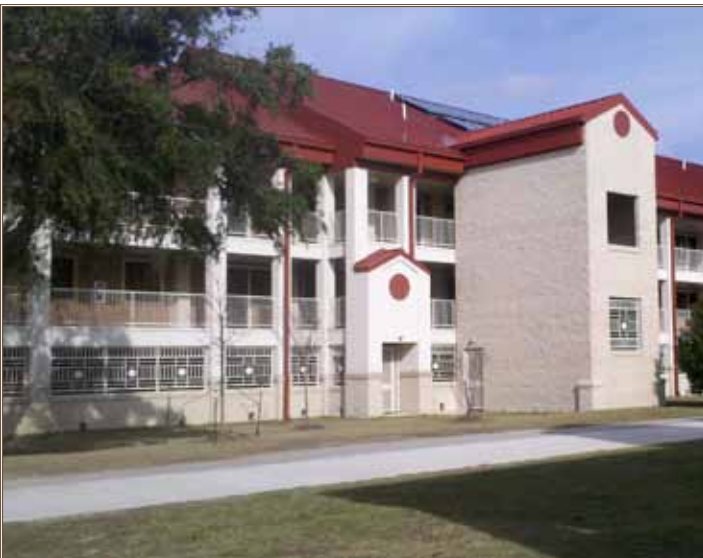
Typical TBUP Barrack exterior with roof mounted solar panels.
