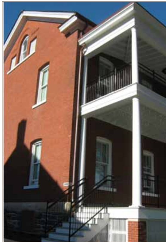
Completed Renovations of Quarters 249, built in 1909, included restoration of original windows on primary façade, as pictured, and reproduction windows on all other façades. Photo by Kristie Lalire, 10Dec12.
