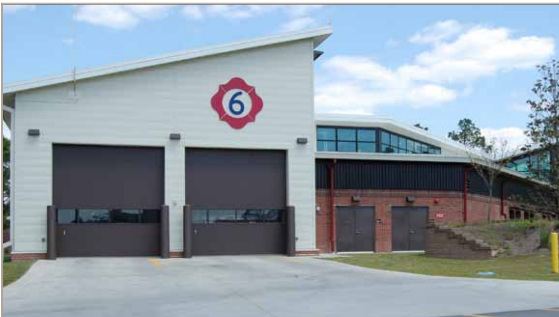
The Linden Oaks CESS demonstrates the efficiency of integrated building design for Army facilities. Completed in March 2011, the project is a combined emergency services facility in a residential community in the Northern Training Area, ten miles north of the main cantonment of Fort Bragg. At 8,295 square feet, the CESS supports a population of 5,500 Soldiers and Family members with fire, emergency services and military police operations.
