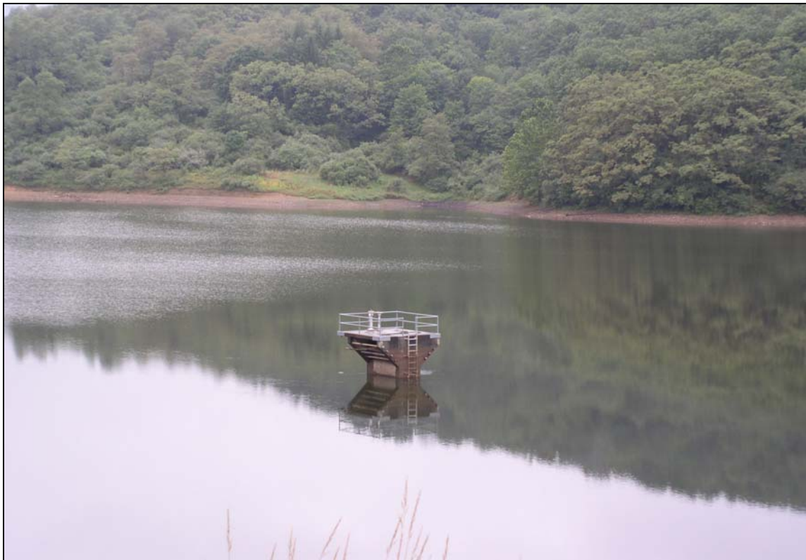
Figure 1 - Existing Riser at NC 14.
