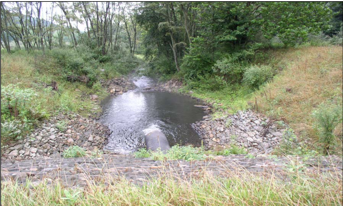
Figure 3 - Outlet Basin Into Linton Creek Below NC 14 Embankment.
