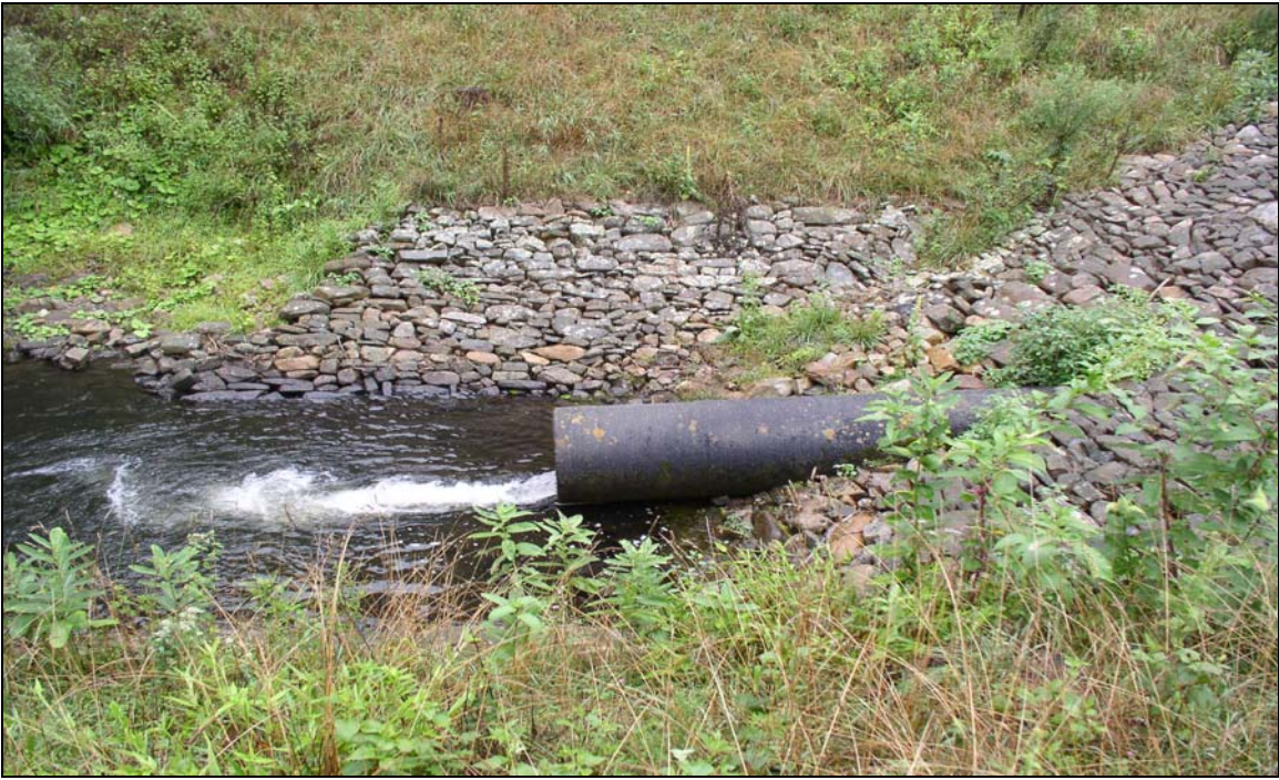
Figure 2 - Principal Spillway Pipe Outlet on Linton Creek Below NC14 Embankment.
