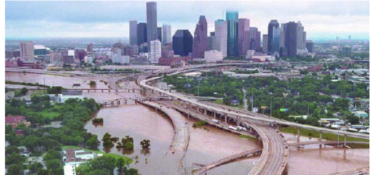
Flooding in Houston during Tropical Storm Allison in June, 2001. More than 35 inches of rain fell in Houston during the storm, killing 41 people and causing more than $5 billion in damage.
