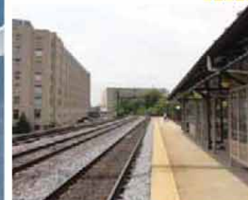
Existing view of the VRE L'Enfant Station platform and CSX Railway.
