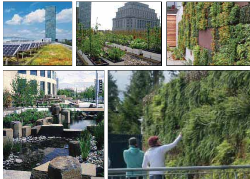
(Images, clockwise from upper left) - Solar/green roof, edible rooftop garden, edible green wall, green wall, rain garden
