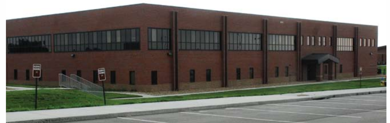
ABOVE AND BELOW: The 1st Sustainment Brigade headquarters building stands tall and fully operational even as the brigade is deployed to Kuwait for 12-months.
