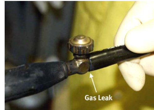
Figure 2-4. Closeup of hose connection at torch valve torch
