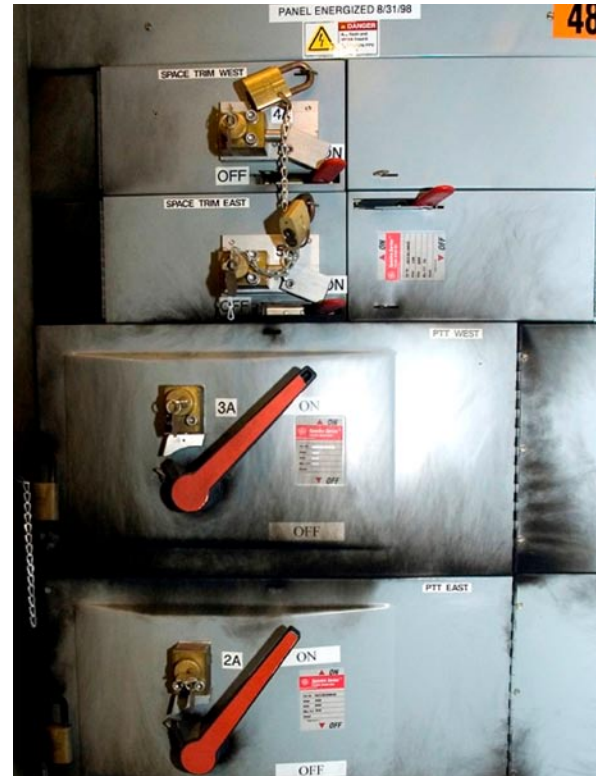
Figure 1-1. Electrical panel PB-1 with switch 3A in the center with signs of arc flash (soot)
