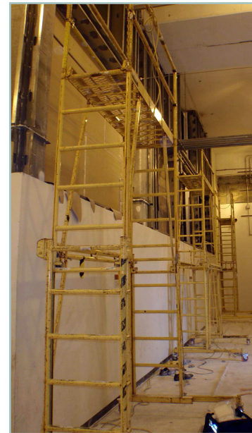
Figure 2-1. Scaffolding in use when accident occurred
