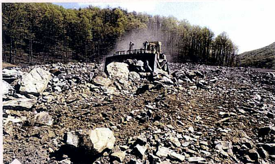
WHITE OAK REFORESTATION RESEARCH PLOTS IN EAST TENNESSEE WHERE AN ALTERNATE GROWTH MEDIA IS BEING LOOSELY GRADED TO FORM A SOIL MEDIUM SUITABLE FOR TREE GROWTH UNDER THE FRA.
