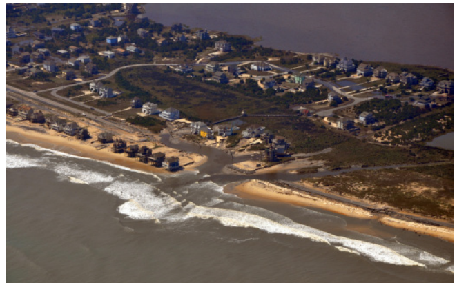
Flooding from Hurricane Irene in August, 2011 sliced through Highway 12 on the Outer Banks of North Carolina. Photo by The Program for the Study of Developed Shorelines, http://psds.wcu.edu
