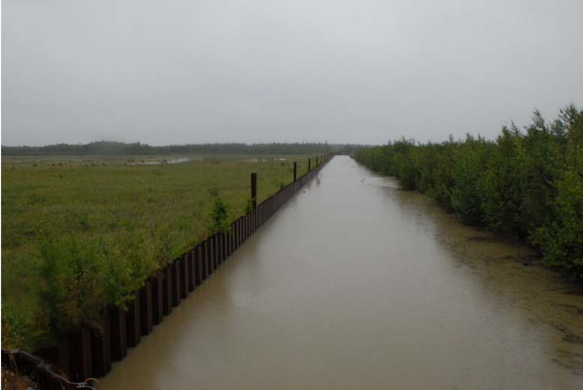
Figure 4. Floodway control sill structure; Tanana River elevation 500.9, July 30, 2009
