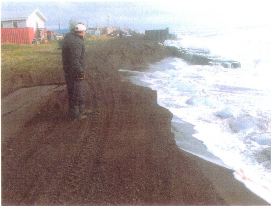
Figure 1. Flanking failure and house on the north end of the existing seawall. (13 Sept, 2007).
